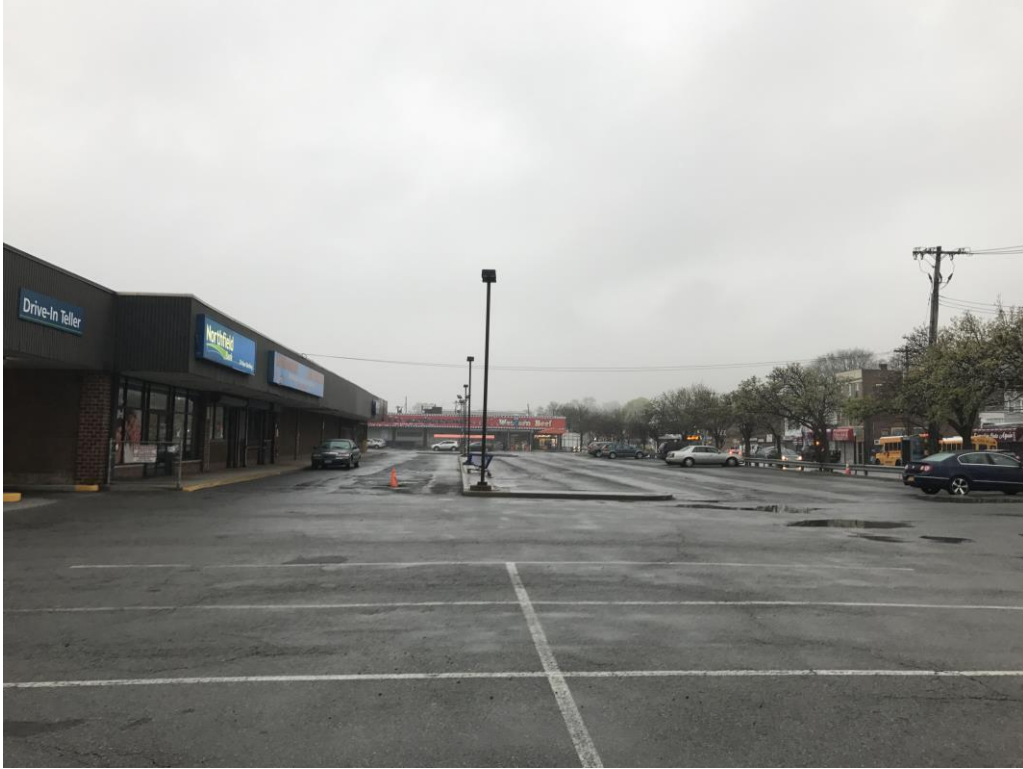
Photograph 3 – View of the parking lot west of the commercial building. Bay Street is visible in the right side of the photograph. Taken facing south.
