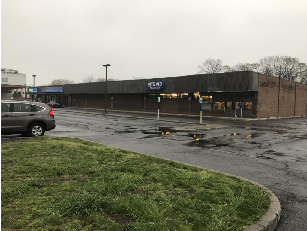
Photograph 1 – View of the south end of the commercial building built in 1984. The building is one story and does not have a basement. Taken facing northeast.
