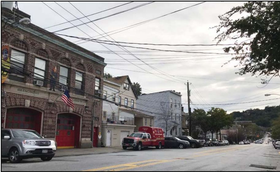
Photograph 1: Looking west on Broad Street from the intersection of Broad Street and Wright Street
