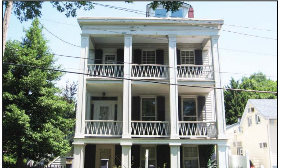
Photograph 8: Mary and David Burgher House on William Street at the intersection of Brewster Street
