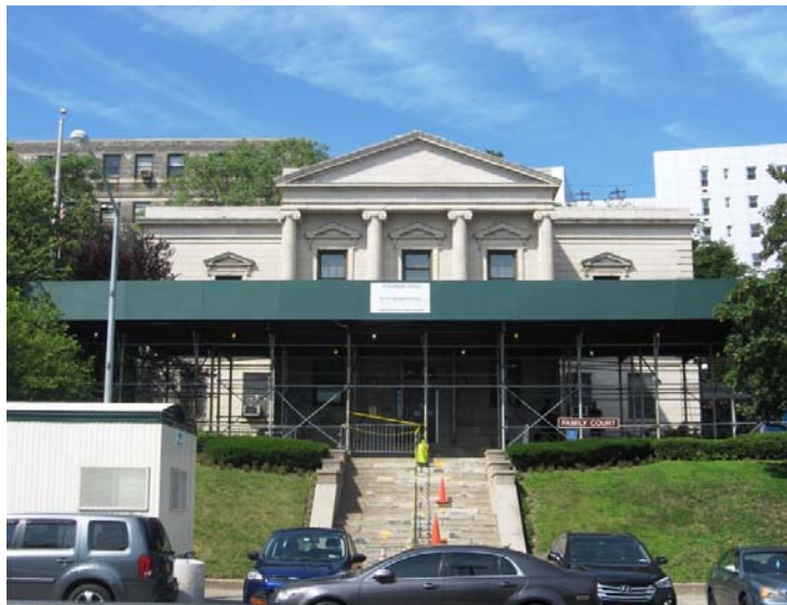
Image 7-3: 120th Police Precinct Station House (LPC-designated, S/NR-Eligible)
