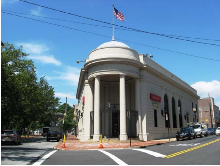
Image 7-10: Staten Island Savings Bank Building (LPC-designated; S/NR-Eligible)
