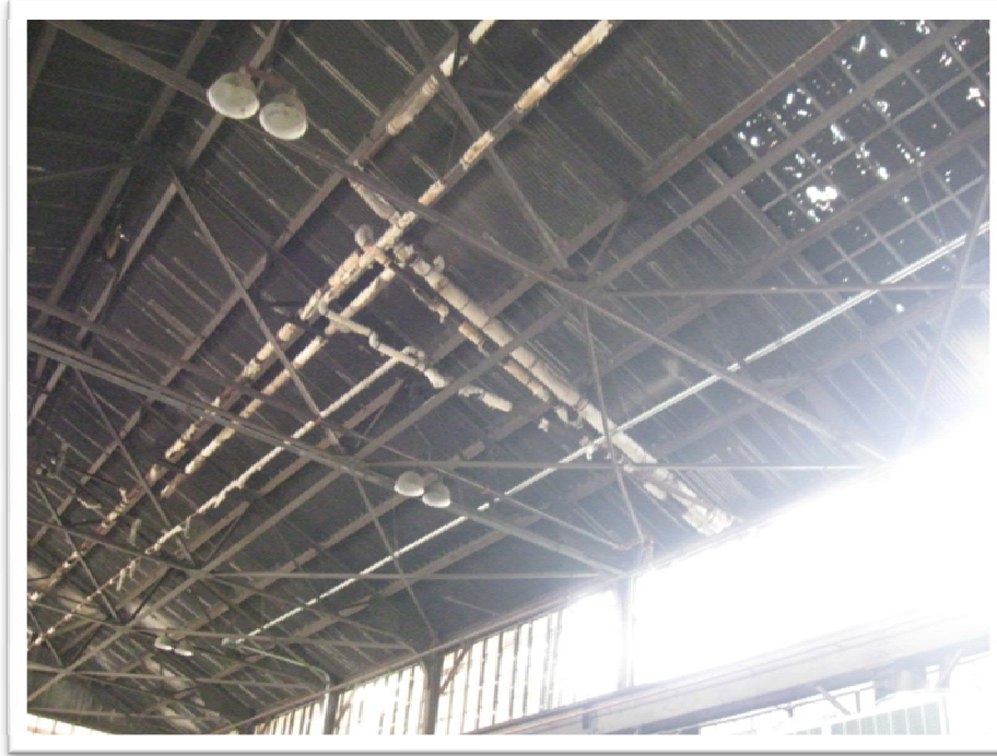
5. Suspect Asbestos- Pipe Chases
