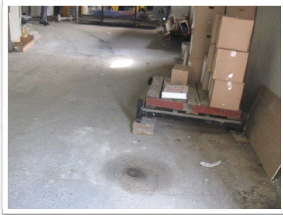
3. Suspect fill pipe inside Building F-Wall Supply Location
