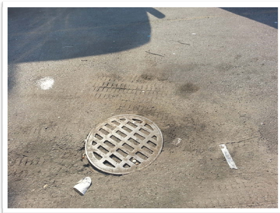
6. Typical Storm Drains of the Site
