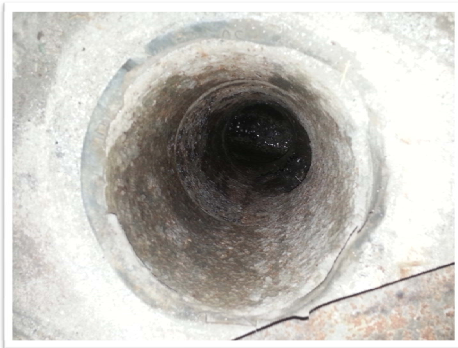
6. Suspect Floor Drains
