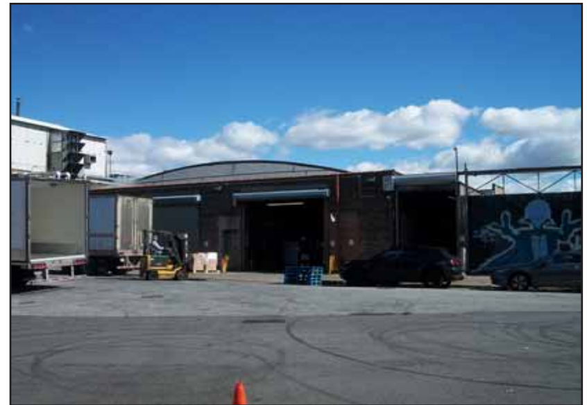
8. Looking north from the intersection of Gem Street and North 15th Street.
