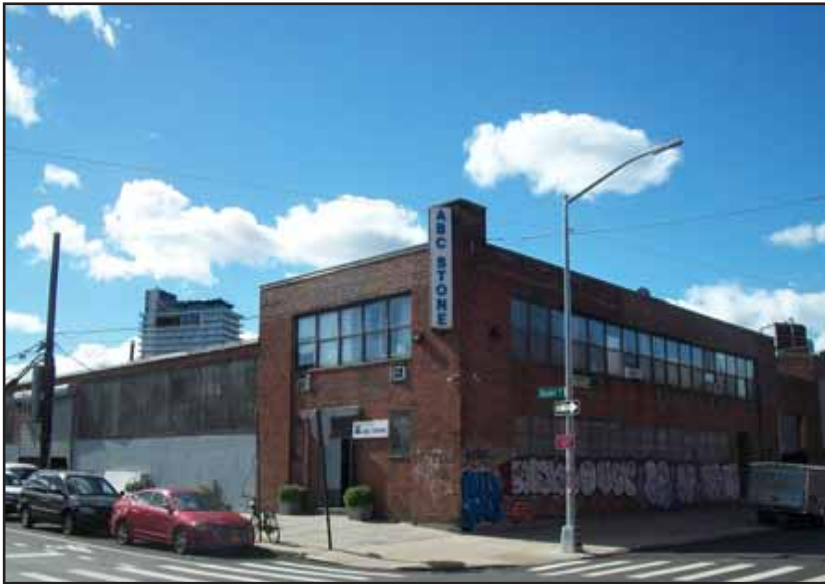
5. Looking southwest from the northeastern corner of the intersection of Banker Street and Meserole Avenue.
