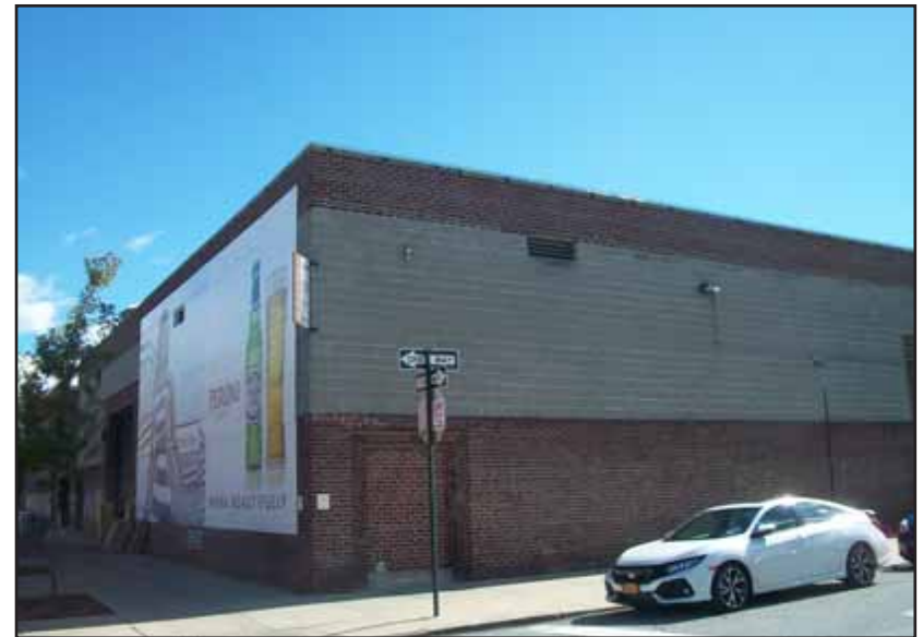
4. Looking southeast from the southwestern corner of the intersection of Gem Street and Meserole Avenue.
