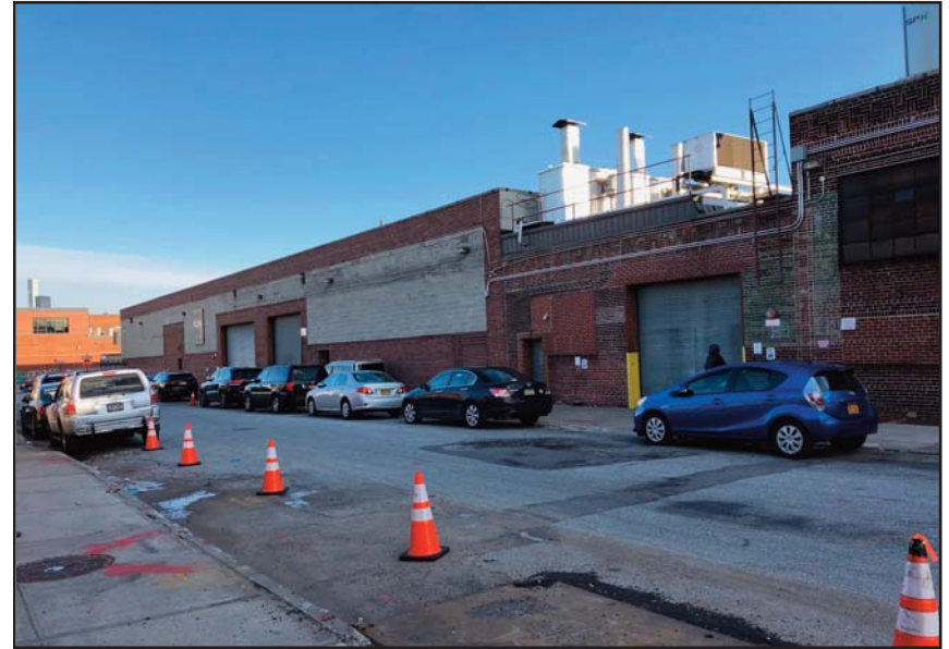
2. View from Gem Street looking northeast towards Acme facility on Lot 1 & a portion of Lot 50.
