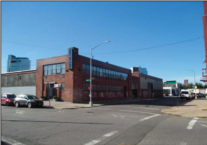
11. View from corner of Banker Street and Meserole Avenue looking southwest towards Lots 6 (left) and 1 (right).
