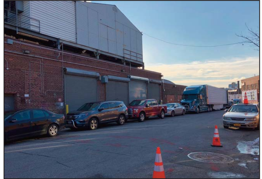
4. View from Gem Street looking southeast towards North 15th Street and Wythe Avenue. Acme facility, with smokehouse on Lot 50, visible to the left.
