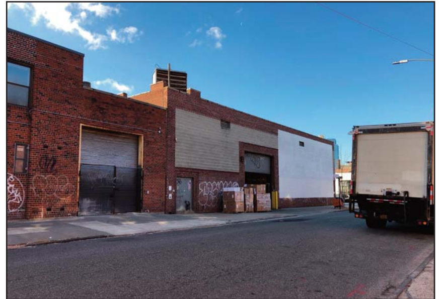
12. View on Meserole Avenue looking southwest towards Acme facility on Lot 1.
