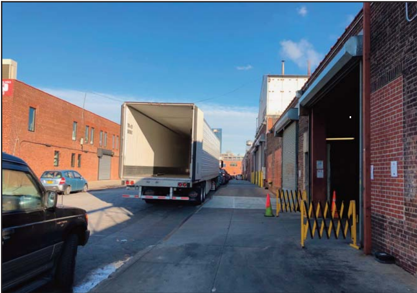
3. View from Gem Street looking northwest towards Acme facility on Lots 21 and 50 (and Lot 1 beyond). Smokehouse on Lot 50 is visible in center right of photo.
