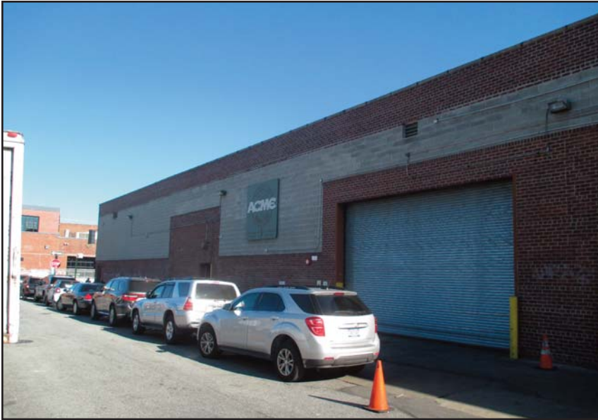
1. View from Gem Street looking northeast towards Acme facility at corner with Meserole Avenue (on Lot 1).
