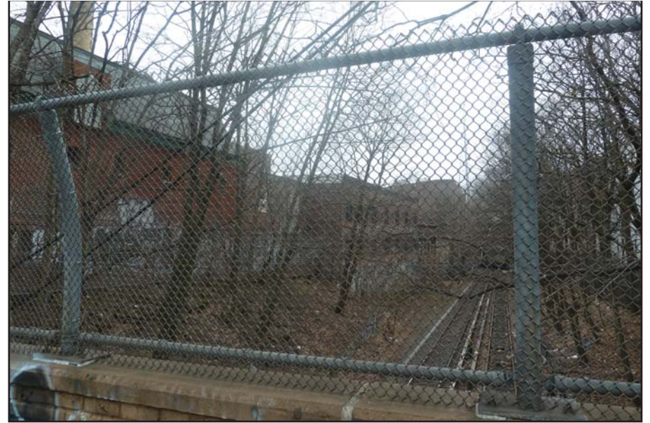
6. View of the Franklin Avenue Shuttle tracks on lot 1 from Montgomery Street, with the existing buildings on the Development Site to the left.
