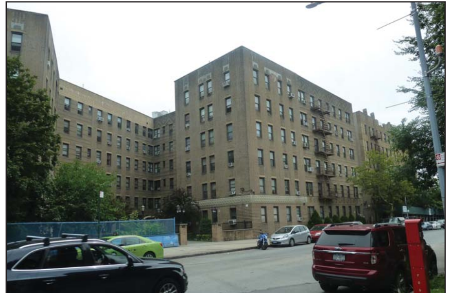
8. View of the apartment buildings fronting Washington Avenue on lots 77 and 85 in the southern portion of the Project Area.
