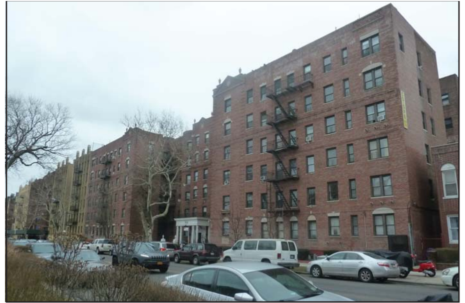
2. Apartment buildings on the south side of Lefferts Avenue between Bedford and Washington Avenues.
