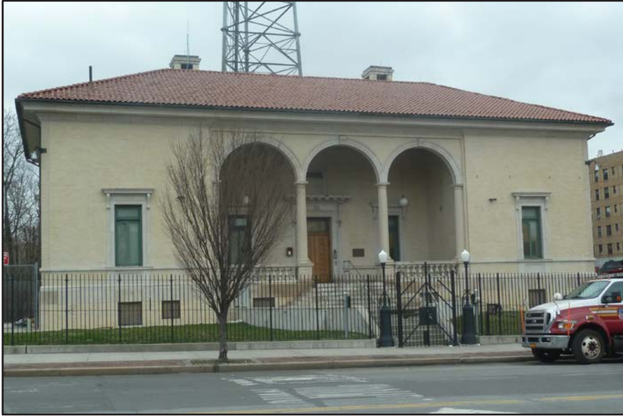
5. View of the LPC-designated and S/NR-eligible Brooklyn Central Office's Bureau of Fire Communication's Empire Boulevard facade.
