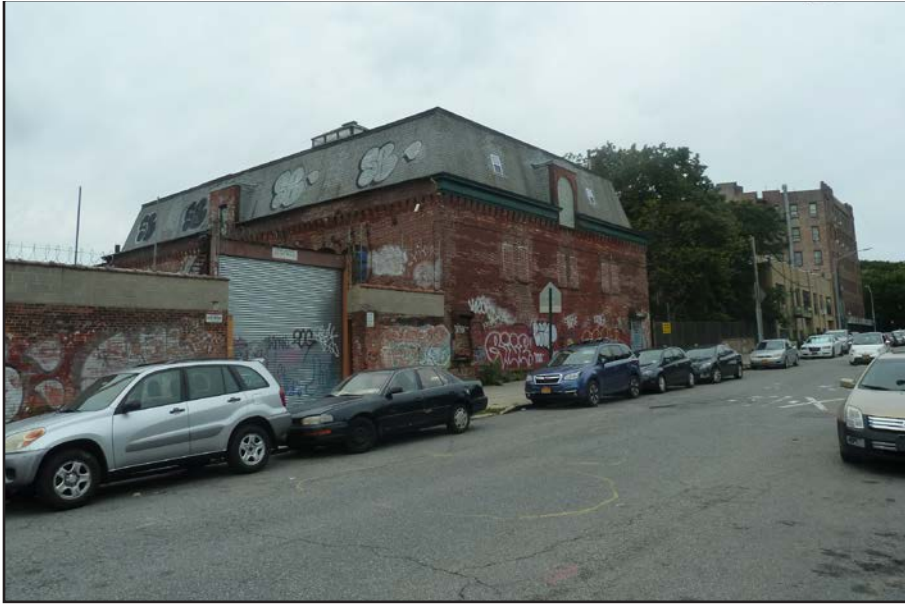
1. View west along Montgomery Street just west of Franklin Avenue, of the former Consumers Park Brewery Complex (S/NR-eligible) stable on Lot 41.
