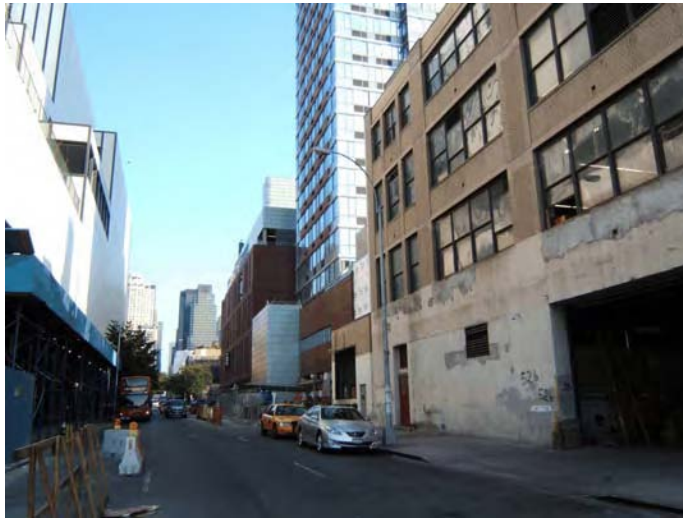
Above: W. 53rd St. south side from midblock toward 10th Ave. TanaSaybert Printing facility (foreground); Archstone Clinton, north tower (mid-ground); Archstone Clinton theatre portion (background)
