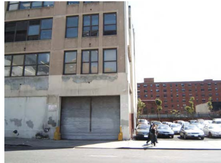
Figure 8-6 Study Area Views: W. 53rd Street South Side, Tenth to Eleventh Avenues
