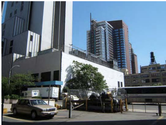
Below: AT&T Switching Tower along W. 54th St. View from Harborview Terrace Houses parking lot on W. 54th St.
