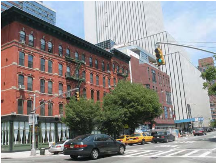
Above: 10th Ave. west side looking north from W. 52nd St. 5-story brick building and low-rise portion of Archstone Clinton; AT&T Switching Tower (background).
