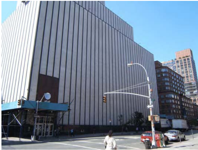
Above: AT&T Switching Tower along 10th Ave. View from 10th Ave. & W. 53rd St.
