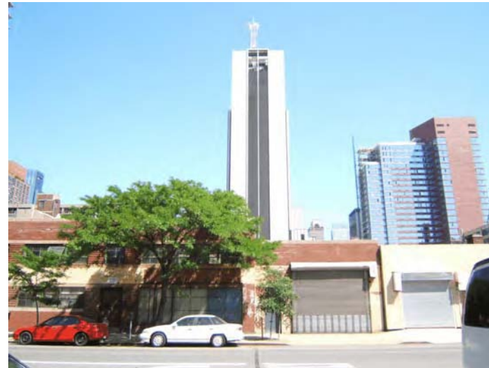
Below: AT&T Switching Tower View from 11th Ave. Project Site in the foreground
