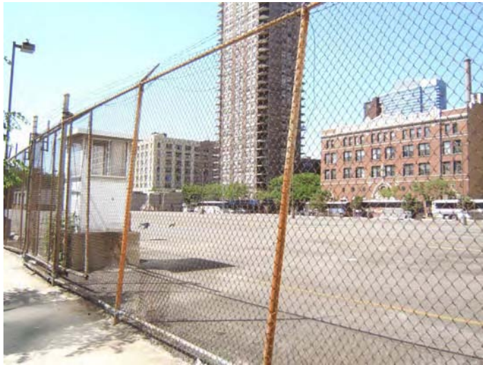
Above: Project Site View from W. 53rd St. Looking Northwest
