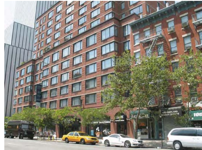
Above: 10th Ave. west side looking south from W. 55th St. 5-story brick building and Archstone West 54th south building; AT&T Switching Tower (background).
