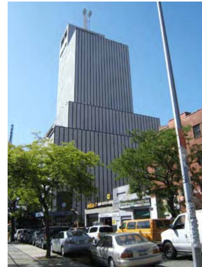
Above: AT&T Switching Tower View from W. 53rd St. East of 10th Ave
