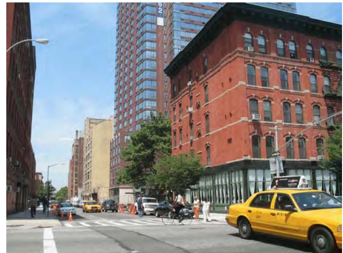
Above: W. 52nd St. south side from 10th Ave. toward midblock. 501 W. 52nd St. (foreground); Archstone Clinton north tower (mid); TanaSaybert Printing building (background).
