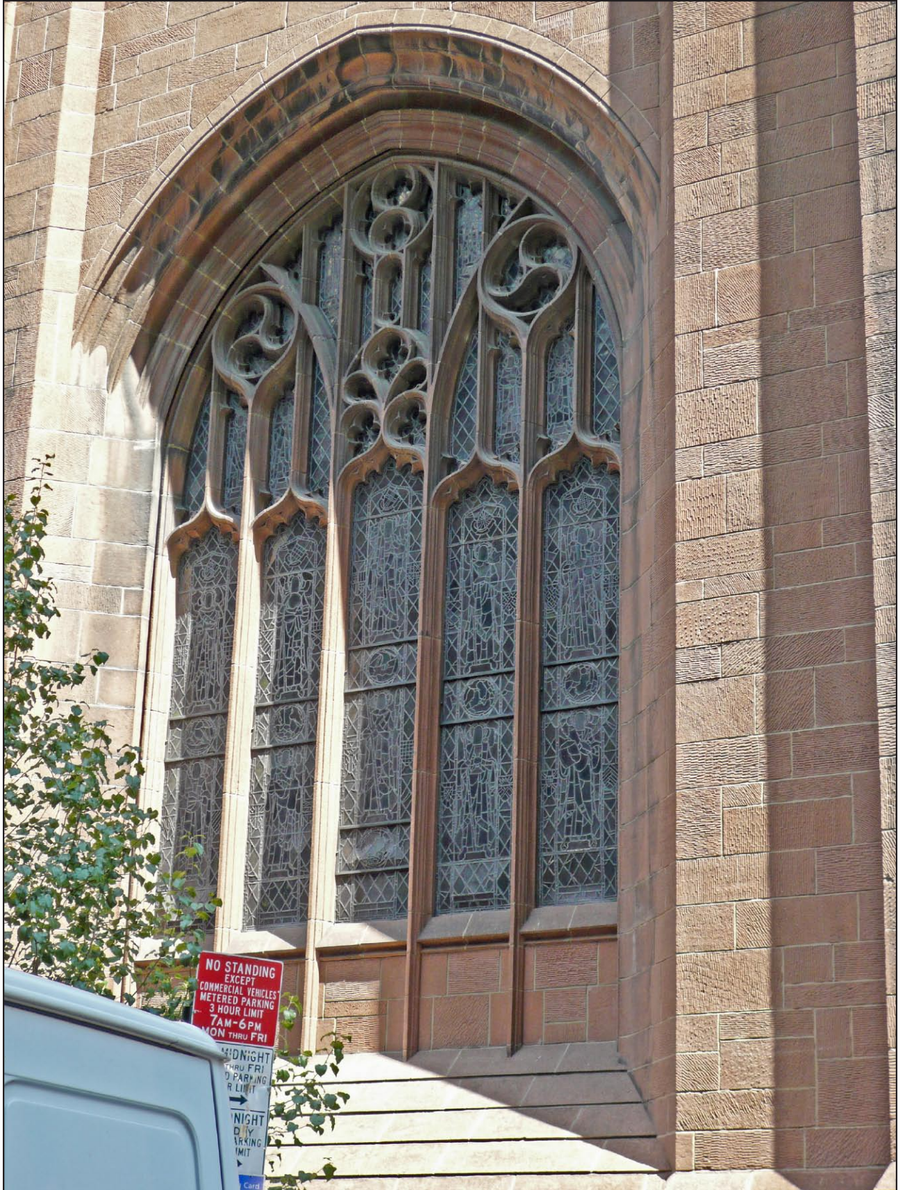
South Window Chapel of Fifth Avenue Presbyterian Church Figure 20-2
