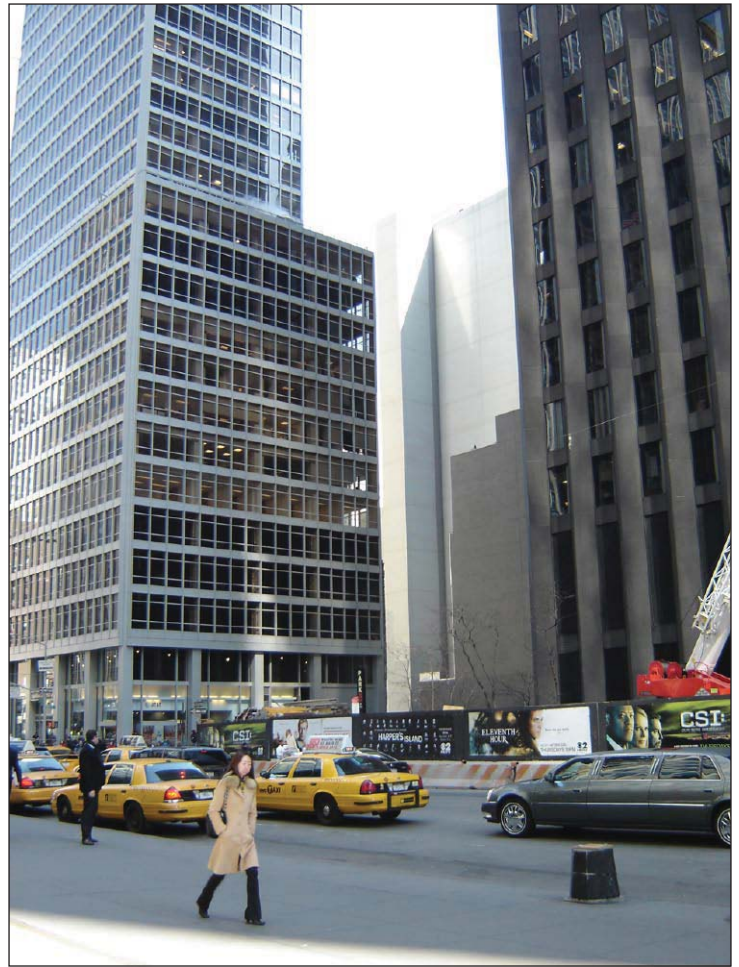
View from Sixth Avenue and West 52nd Street to development site 21
