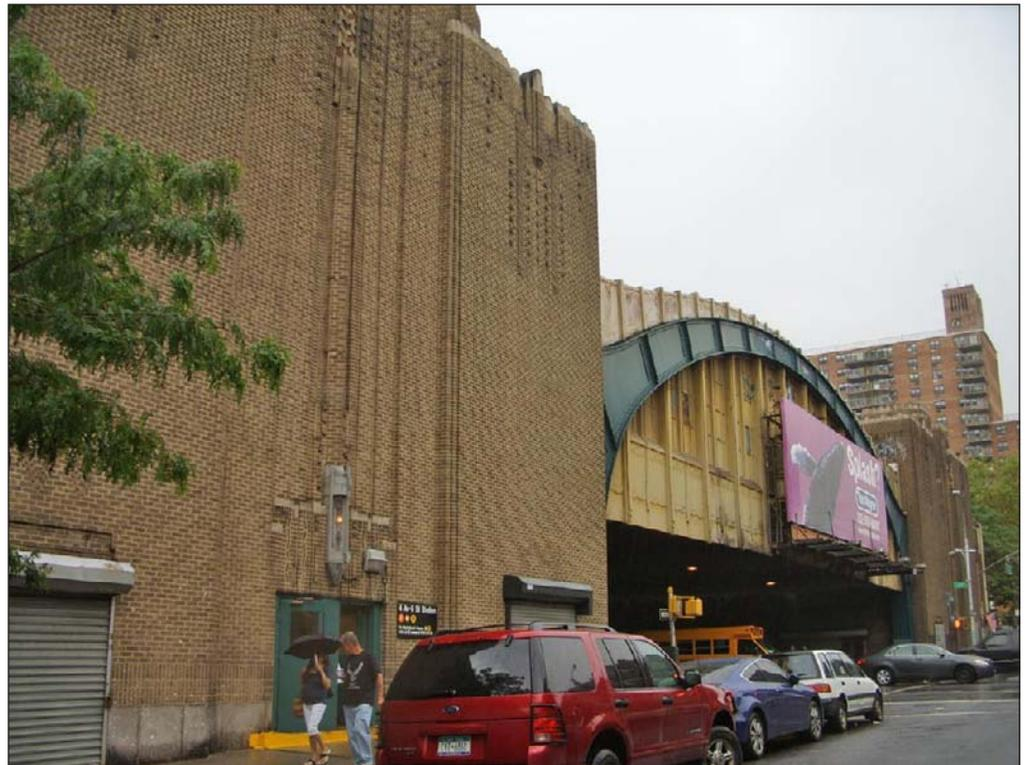
Looking northeast from 10th Street and 4th Avenue to the IND subway viaduct where it crosses 4th Avenue. This portion of the viaduct, consisting of a steel-arch and brick piers designed in the Art Deco-style, houses the 4th Avenue subway station, which is listed on the S/NR
