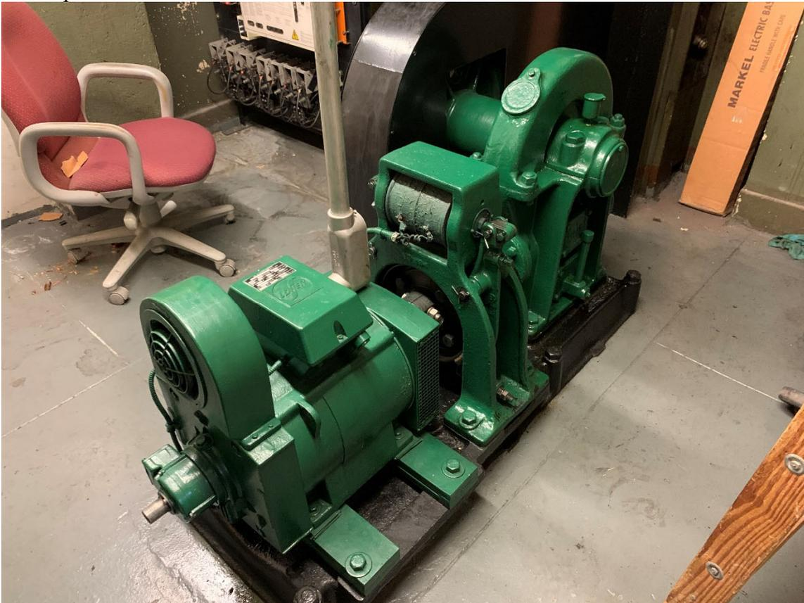
Photograph No. 17: A typical cable-operated elevator mechanical room observed within Lot 48.
