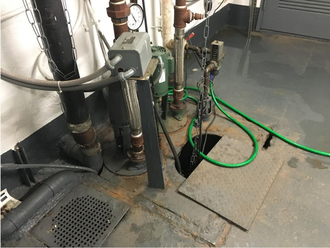
Photograph No. 16: An existing sump pit associated with floor drains, piped into the municipal sewer.
