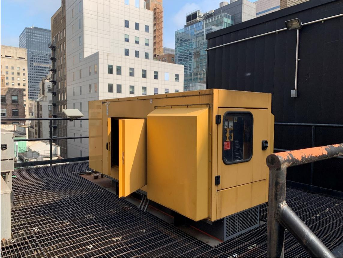
Photograph No. 13: An existing rooftop diesel-fired emergency backup generator associated with Lot 23.
