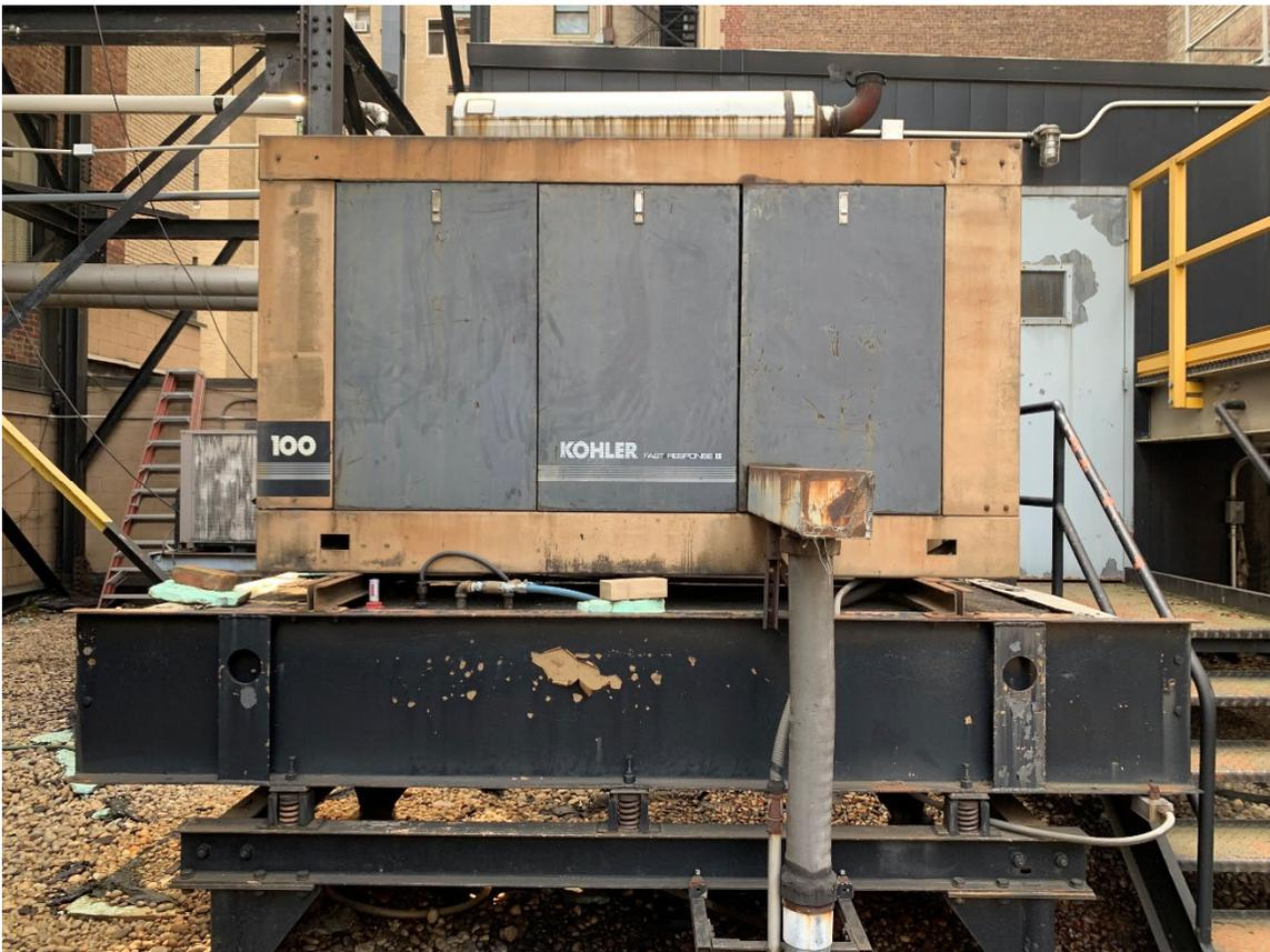
Photograph No. 14: An existing rooftop diesel-fired emergency backup generator associated with Lot 23.
