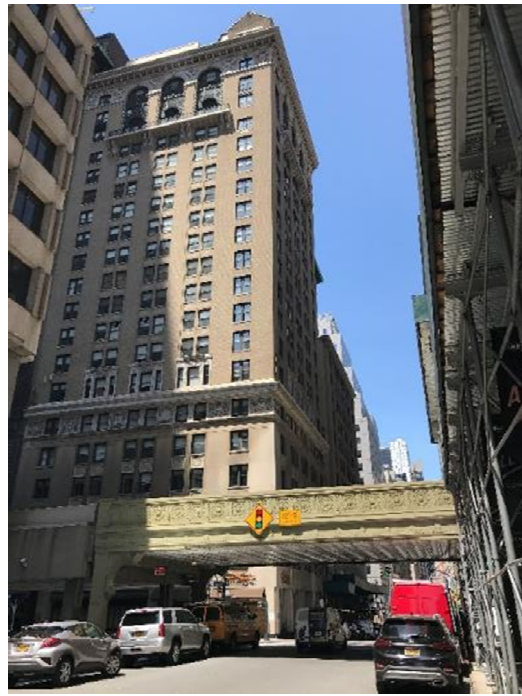
Photo 6-4 View of 52 Vanderbilt Avenue west along East 45th Street
