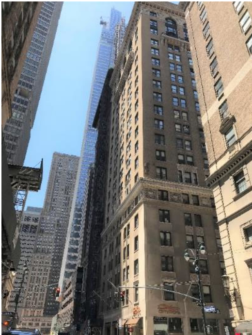
Photo 6-7 View south along Vanderbilt Avenue from 45th Street
