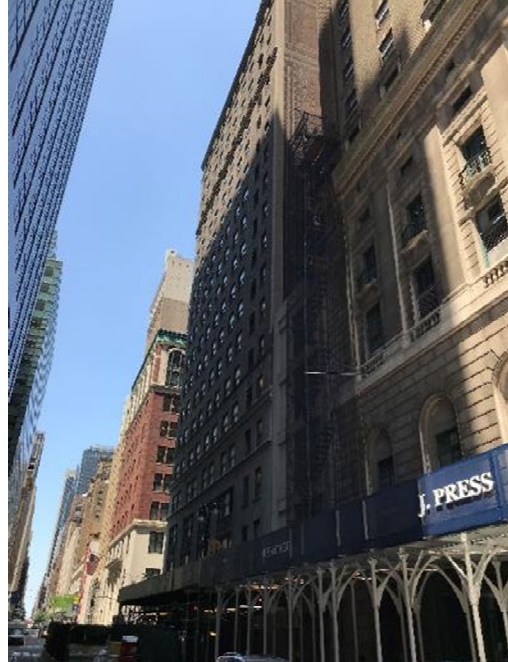
Photo 6-2 View of Project Site facing west along East 44th Street
