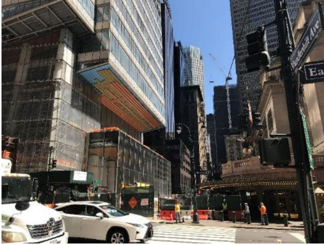
Photo 6-13 Pedestrian plaza adjacent to One Vanderbilt currently under construction
