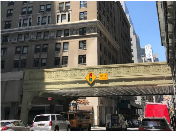
Photo 5-7 East 45th Street Bridge (portion of Park Avenue Viaduct)
