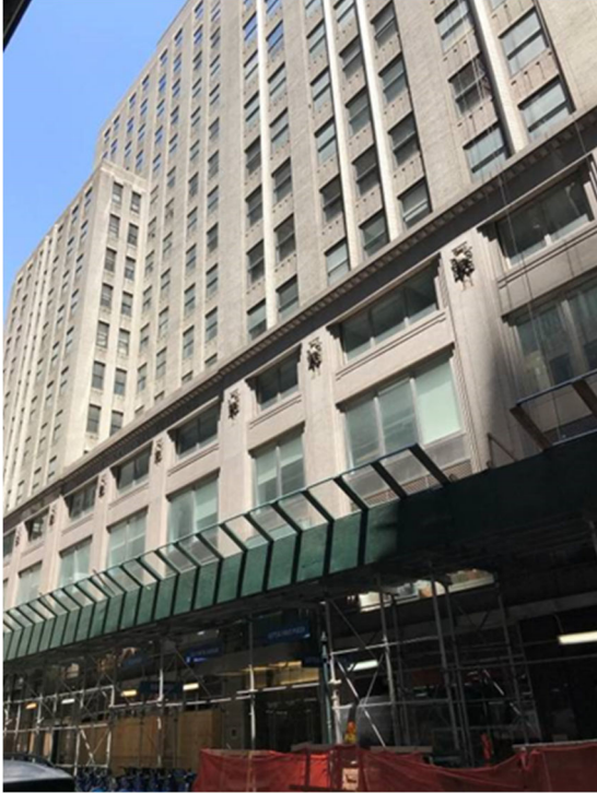
Lefcourt-National Building (#9). View northwest on East 43rd Street
