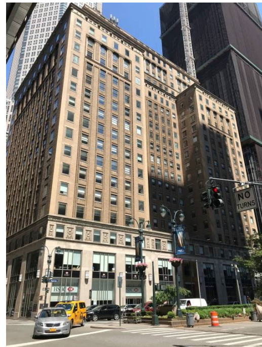
Postum Building (#8). View northwest on Park Avenue
