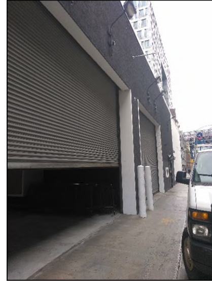
Photograph 6: Bay doors along the western side of 307 Kent Avenue.
