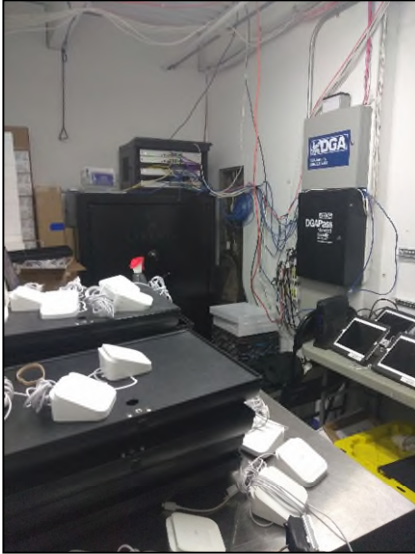
Photograph 5: Lofted office space on the mezzanine level of 307 Kent Avenue.
