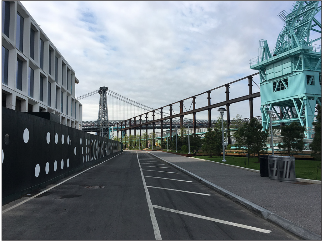
River Street, view south from north end of Domino Park 15
