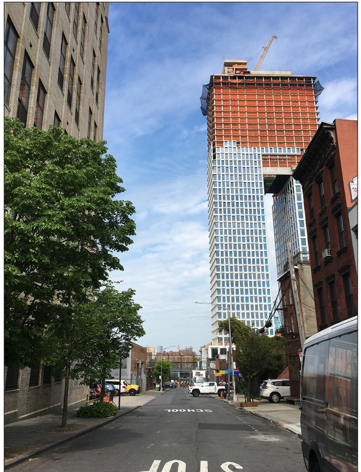
South 1st Street, looking west from Wythe Avenue 18
