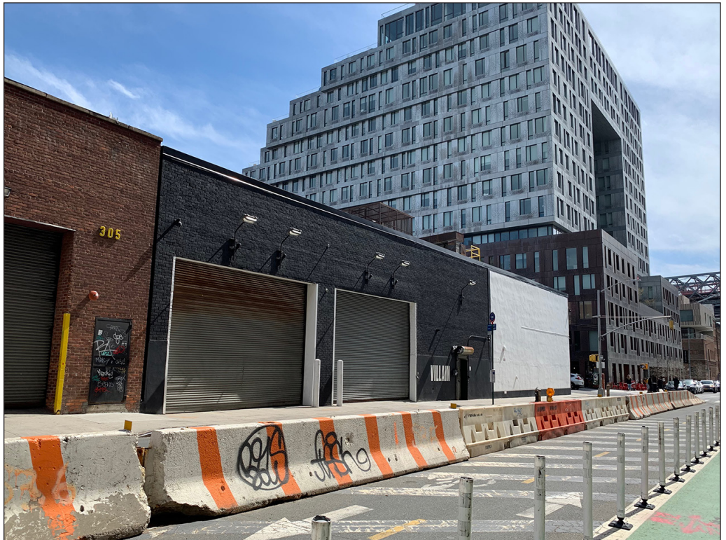
View of Projected Development Site 1, looking southeast from Kent Avenue 1
