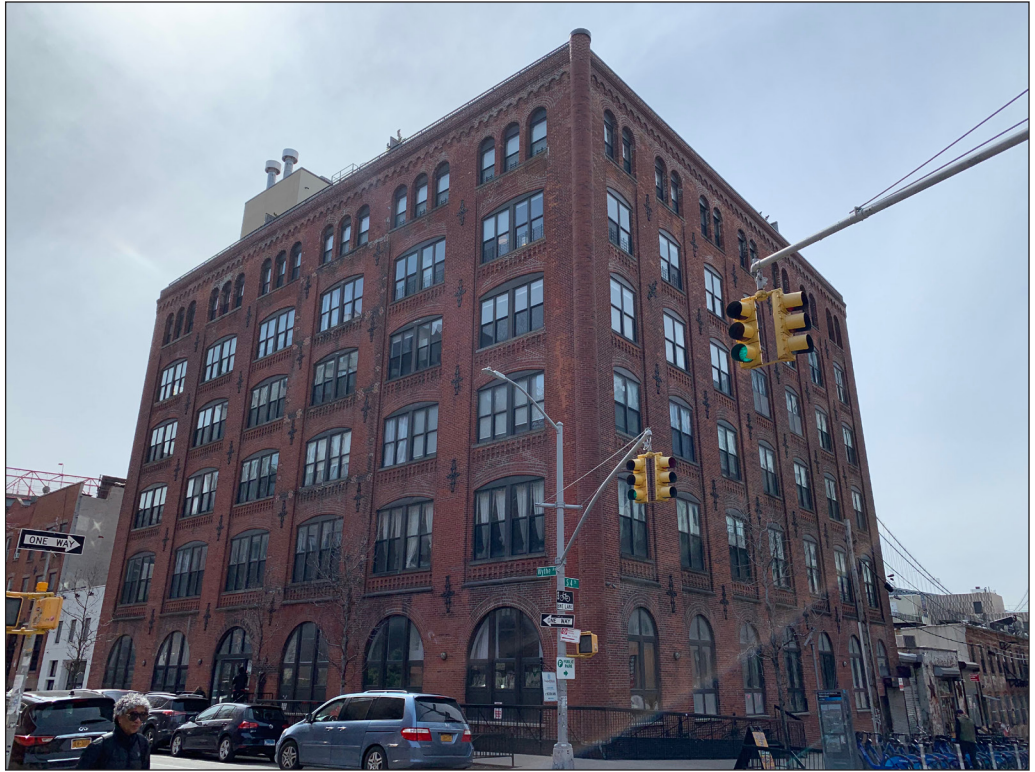
Former Matchett Candy Factory building, view southwest from Wythe Avenue and South 4th Street 13
