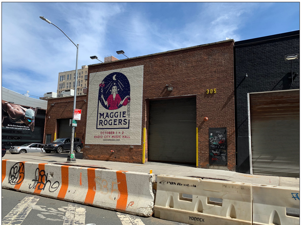
View of Projected Development Site 2, looking east from Kent Avenue 2
