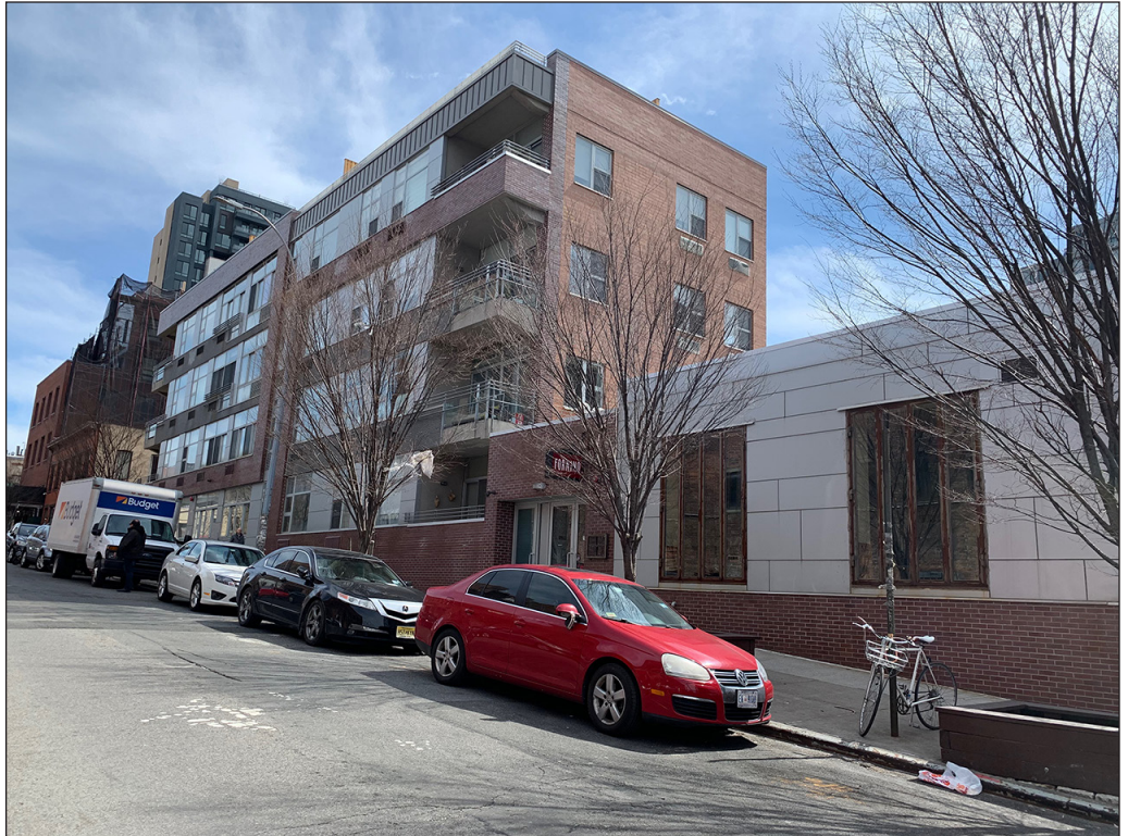
View of development on Lots 10 and 7502, looking east on South 2nd Street 3
