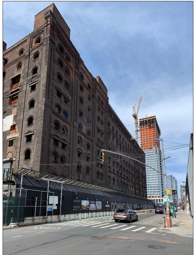
Former Havemeyers & Elder Filter, Pan & Finishing House, view north on Kent Avenue 8
