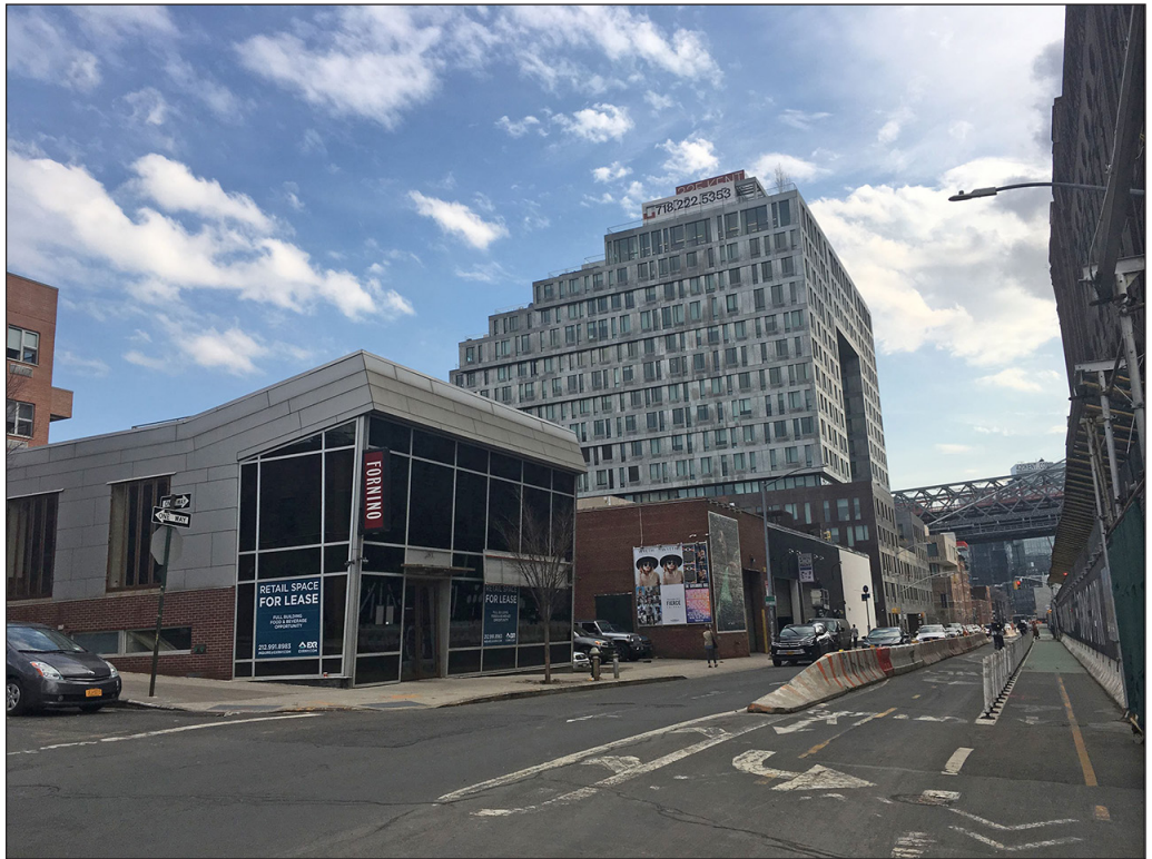
View southeast along Kent Avenue from South 2nd Street showing Projected Development Site 2 and Projected Development Site 1 6
