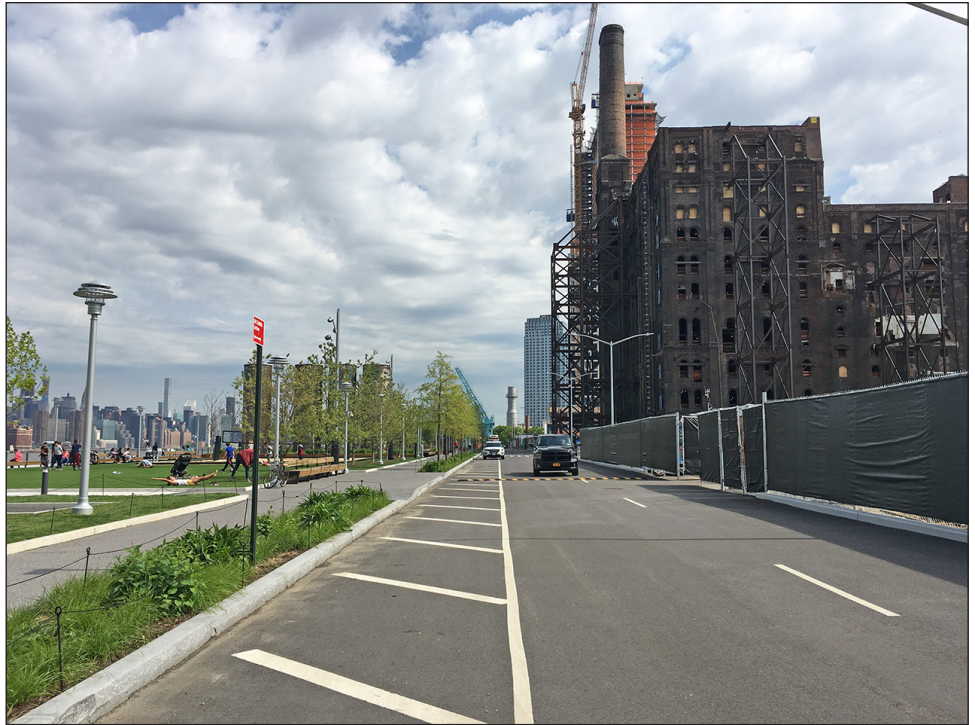
River Street, looking north from South 4th Street 17
