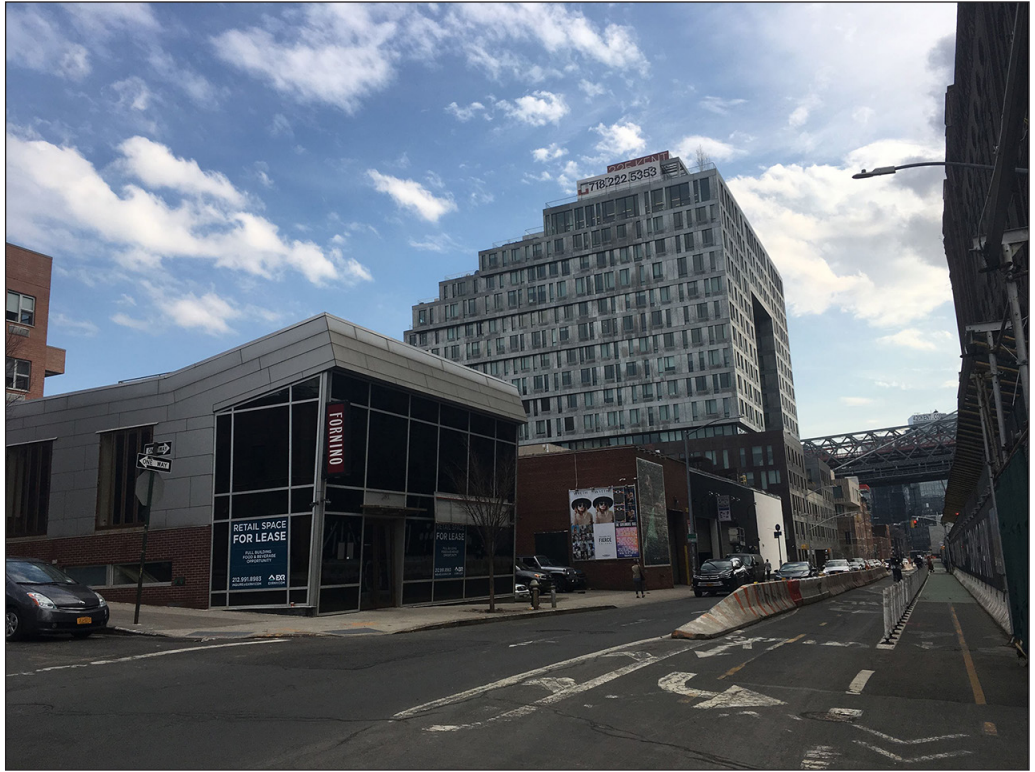
Project Area, view southeast from Kent Avenue at South 2nd Street 7
