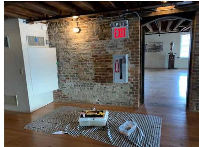
Photograph 4: Typical room refinished for museum display purposes on the 5 th Floor of 93 South Street/2 Fulton Street.
