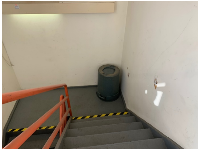
Photograph 11: Typical stairway in 167-171 John Street.
