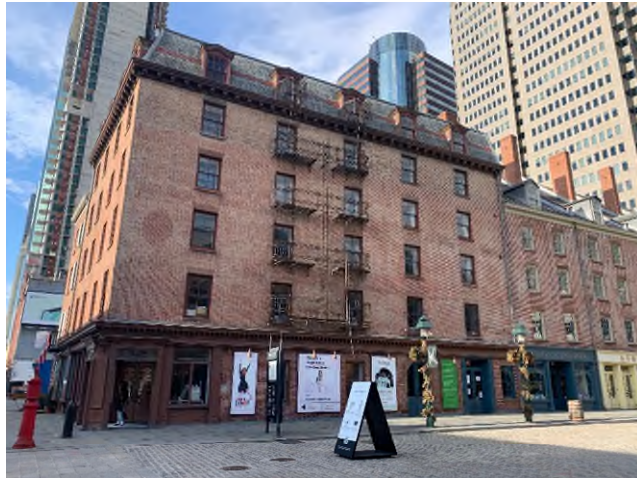
Photograph 1: Building exterior of 93 South Street and 2-4 Fulton Street as seen from Fulton Street.
