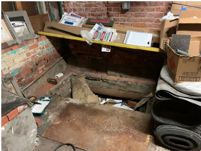
Photograph 7: Sump pit in the basement of 167-171 John Street.
