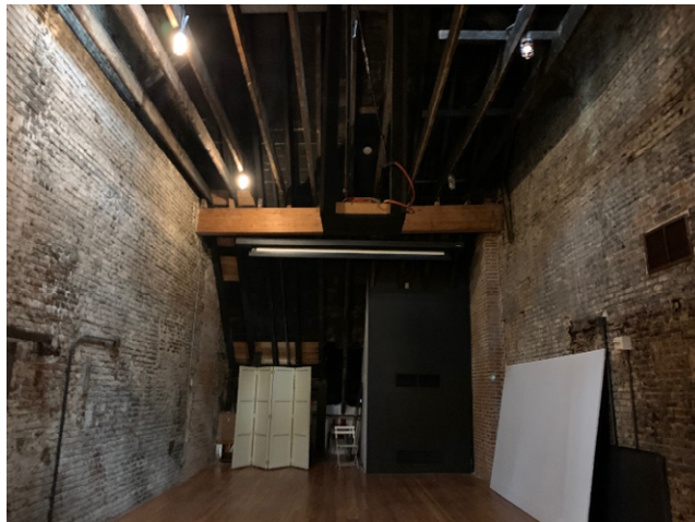
Photograph 3: Typical interior room used for museum storage on the 5 th Floor of 91 South Street.
