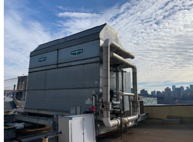
Photograph 10: Air handler on the roof of 167-171 John Street.
