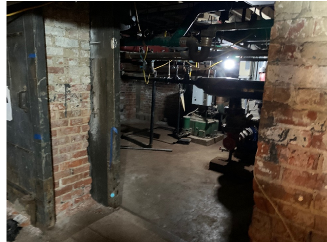
Photograph 6: 167-171 John Street basement mechanical space.
