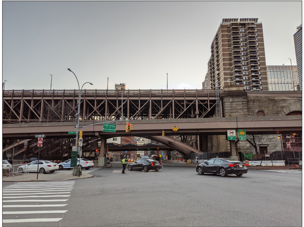
View west on St. James Place 27
