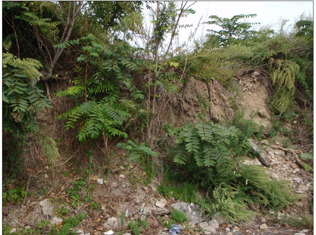
Eroding, mixed-fill, solid waste berm on the northwest shoreline of project site 11
