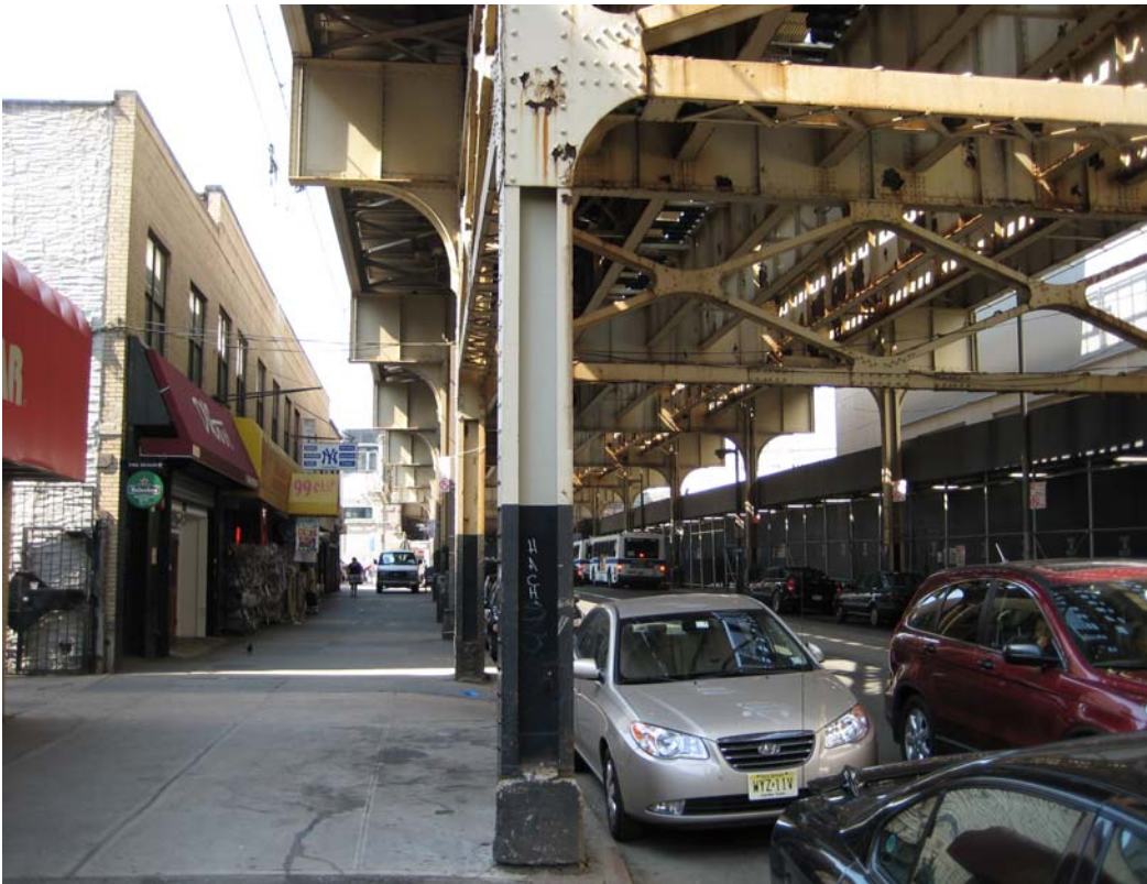
(2) A view of the elevated train and River Avenue, facing south
