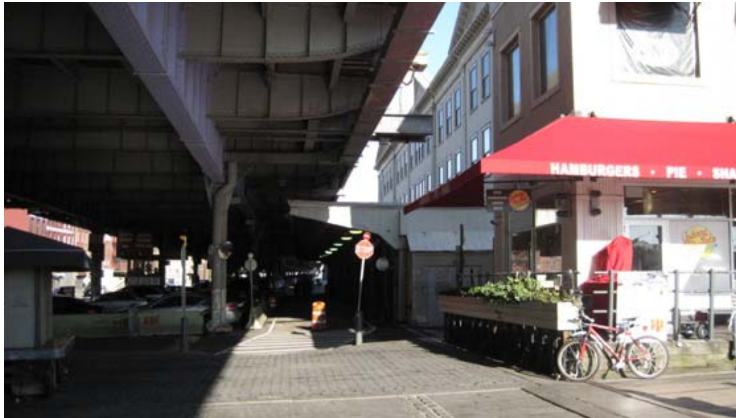
03 VIEW NORTH ALONG SOUTH ST. LINK BUILDING IN FOREGROUND
