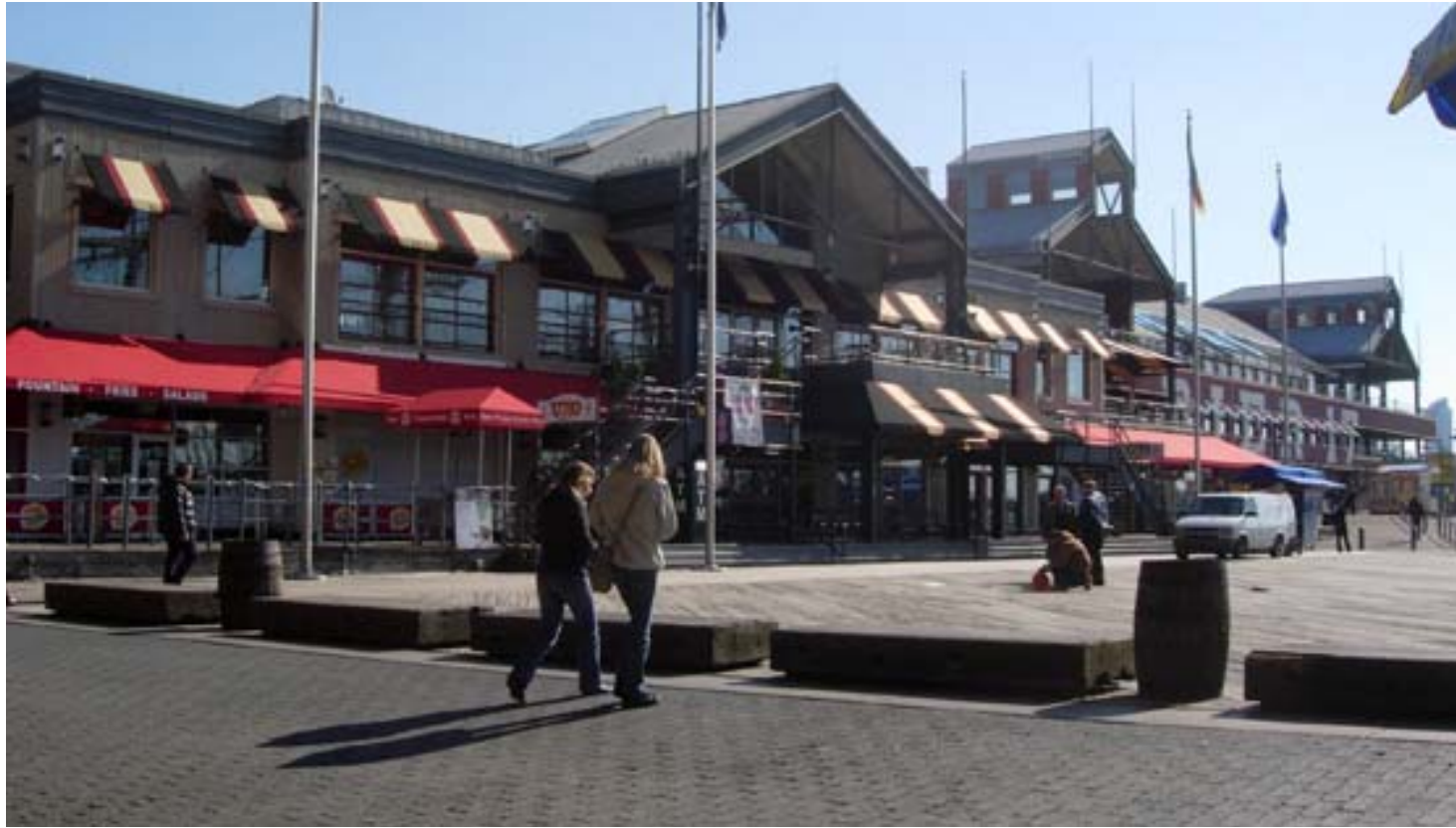
01 VIEW NORTH ALONG SOUTH STREET SHOWING LINK BUILDING IN FOREGROUND
