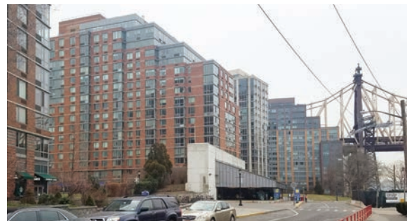
Building in a non-contextual district
