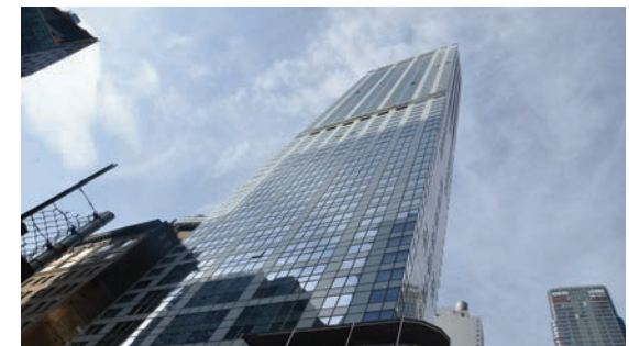
Building using tower regulations
