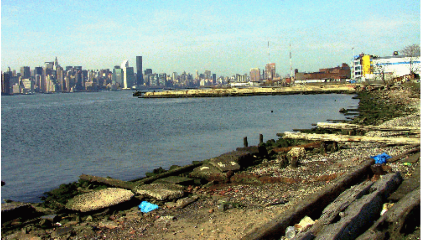
WILLIAMSBURG WATERFRONT 197-a PLAN (2002): Portion of former Eastern District Terminal acquired by the state for a new park with playing fields and an esplanade.
