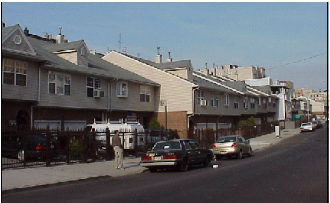
MORRISANIA 197-a PLAN (1992): New York City Housing Partnership homes constructed since adoption of the plan.
