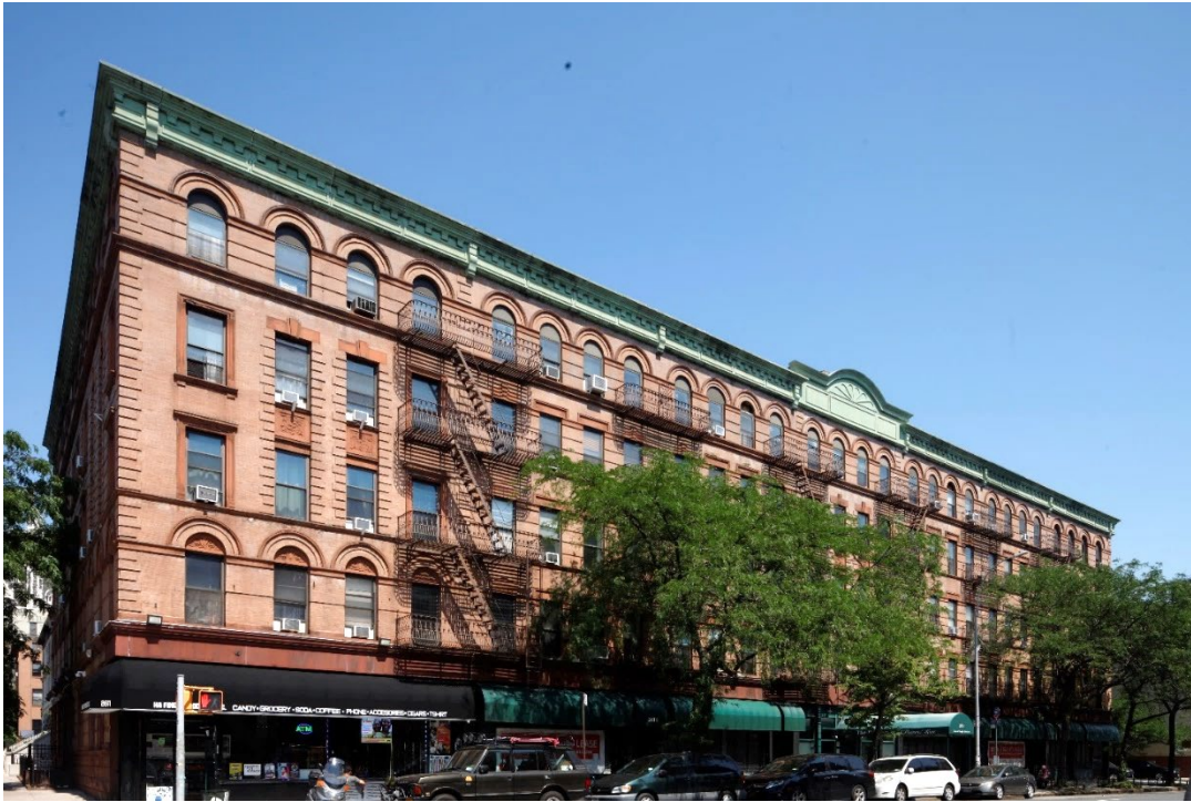
Figure 5 2611 through 2623 Frederick Douglass Boulevard Jessica Baldwin, LPC, 2021
