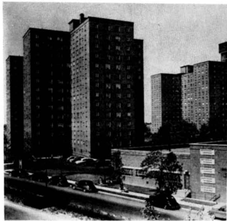
PARKING SPACE AND PARKING GARAGE IN A LARGE-SCALE RESIDENTIAL DEVELOPMENT.
