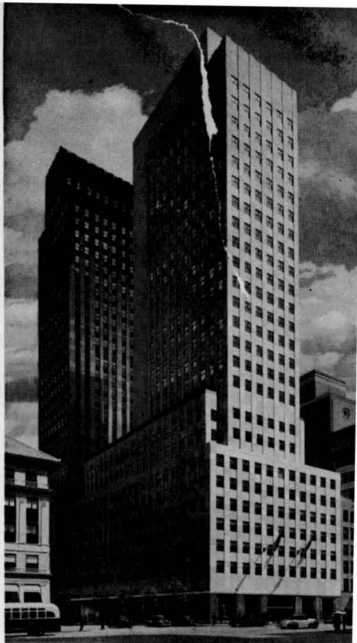
OFFICE BUILDING DESIGNED FOR MAXIMUM LIGHT AND Practical elimination of setbacks confines most of the structure a fourth of the lot area, making it impossible for future buildings to cut off light, view and air. 600 Fifth Avenue. Carso Lundin, Architects.
