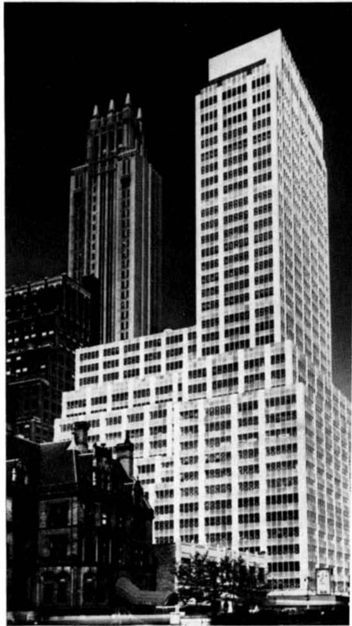
CURRENT HIGH BULK OFFICE CONSTRUCTION. Illustrative of current construction in the Grand Central Area proposed for Commercial A-4 is the building at 100 Park Kahn and Jacobs, Architects.
