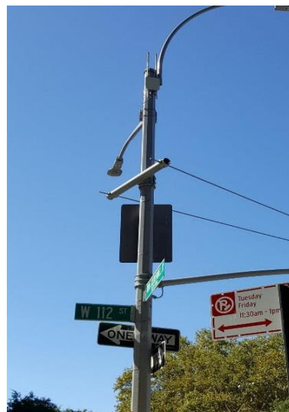
Image 2: A Wi-Fi access point attached to a street pole on West 112th Street in Harlem.
