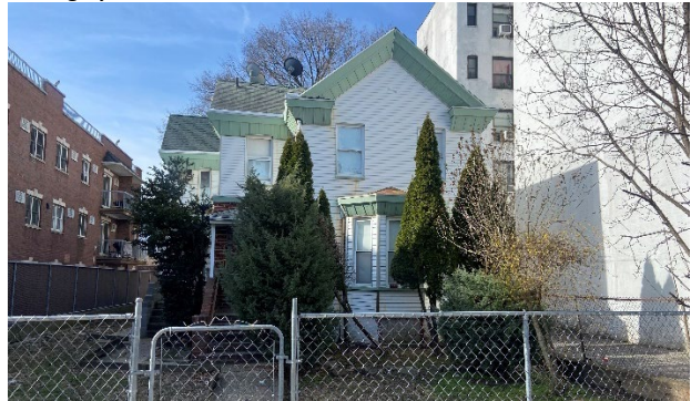
View south from Ovington Avenue to Projected Development Site 1. The site contains a 2-story, two-family residence.
