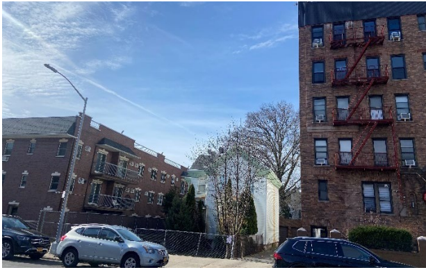
View south across Ovington Avenue to Projected Development Site 1. 460 Ovington Avenue is shown on the right (5-story residential building), and 474 Ovington Avenue (3-story mixed-use residential and community facility building).
