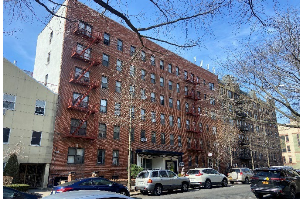
View west across Ovington Avenue towards 420 Ovington Avenue, a 6-story multifamily building that abuts the Proposed Rezoning Area. 428 Ovington – shown in the far left of the frame – is in the Proposed Rezoning Area.
