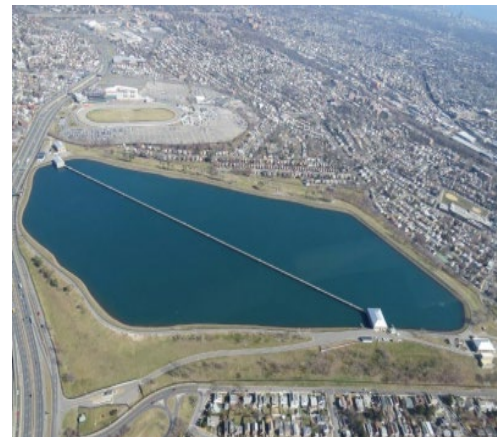
Figure 7-5: Hillview Reservoir Located in Yonkers
