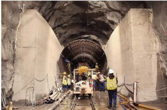
Figure 7-6: Delaware Aqueduct By-pass Tunnel Triple Pass Design
