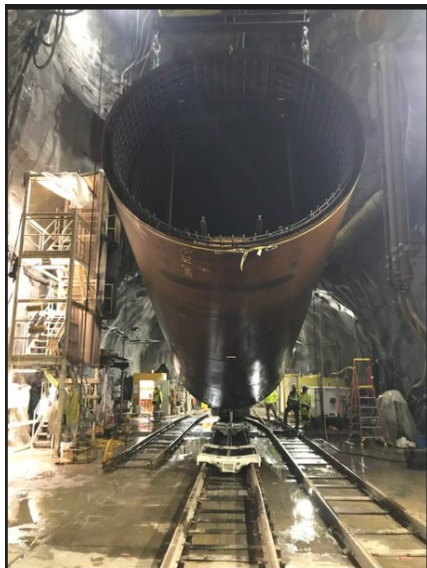
Figure 7-5: Delaware Aqueduct By-pass Tunnel Installation of Steel Liner
