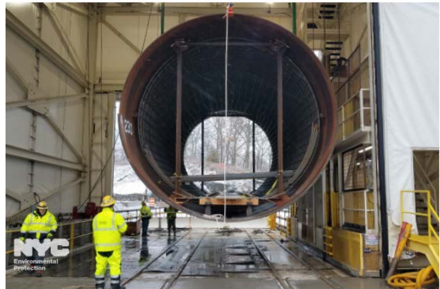
Figure 6-6: Delaware Aqueduct by-pass tunnel installation of steel liner
