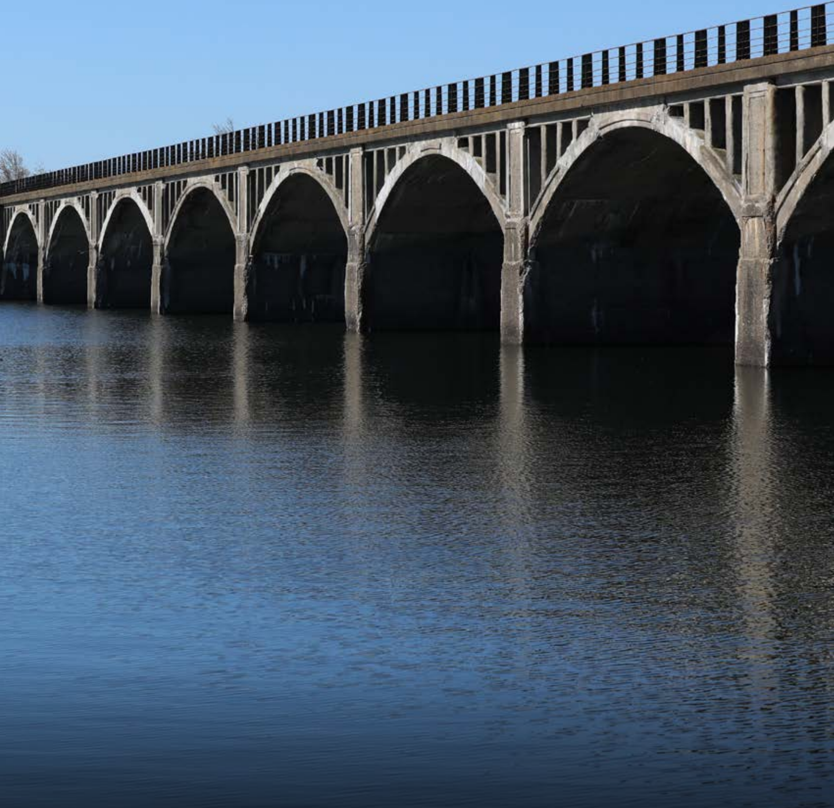
Dividing Weir bridge at Ashokan
