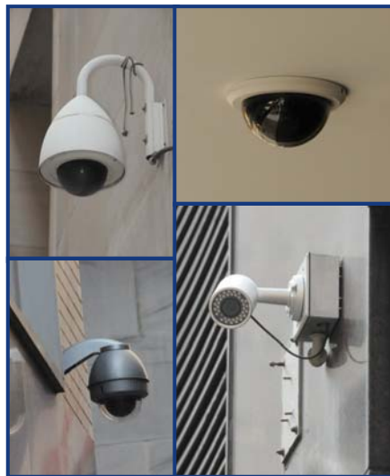
CCTV cameras in many shapes and sizes.
