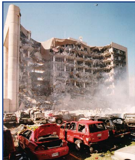
Alfred P. Murrah Federal Building, Oklahoma City 1995
