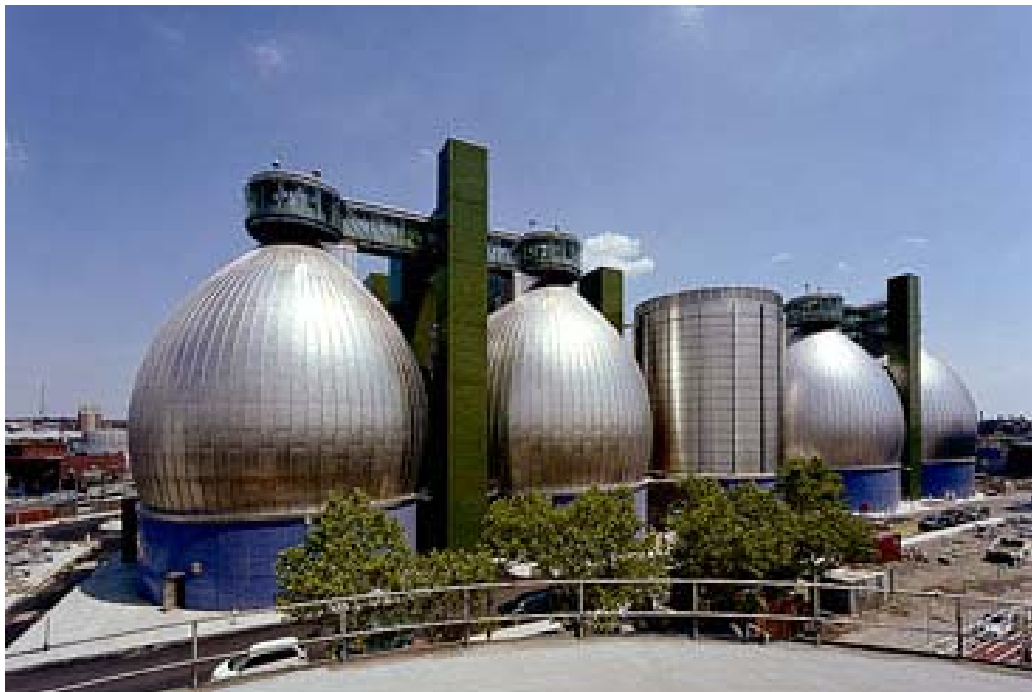
Newtown Creek Wastewater Treatment Plant Digester Eggs
