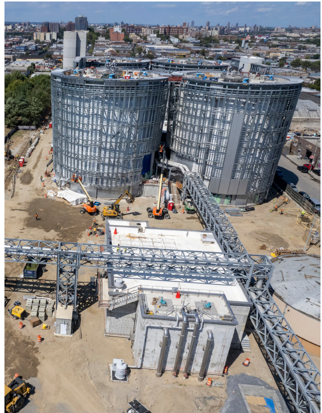
Hunts Point digesters construction project
