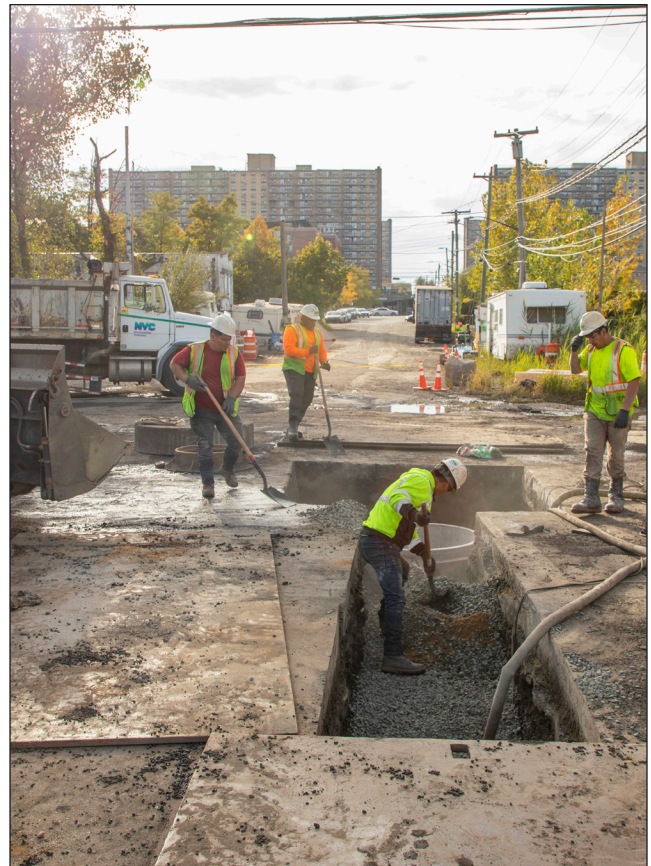
Sewer upgrade project, Jewel Street neighborhood, Brooklyn
