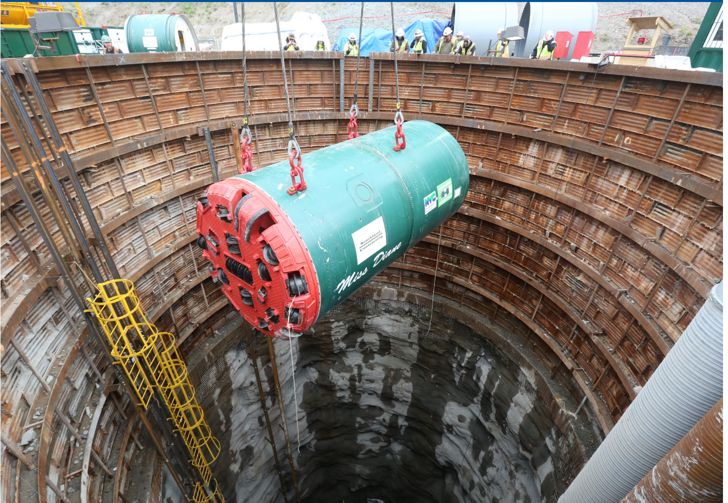
Micro-tunneling machine at Schoharie Reservoir
