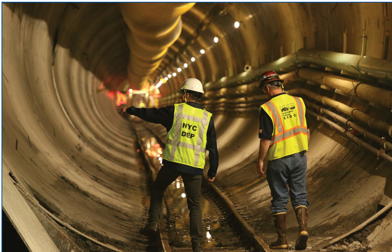
Delaware Aqueduct Bypass Tunnel
