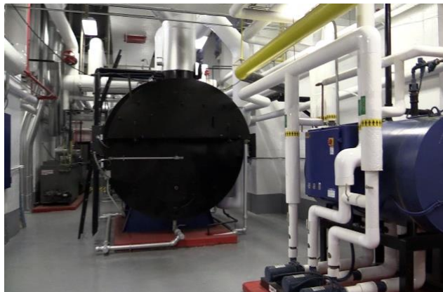
New and improved building systems at Ocean Bay (Bayside)
