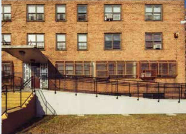
View of entry to commercial spaces
