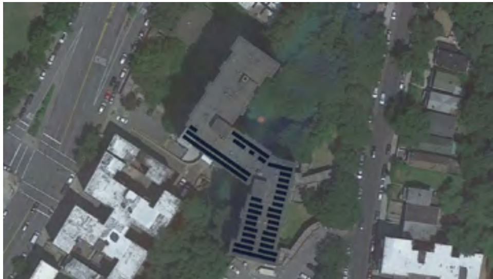
Fort Independence Solar PV Potential
