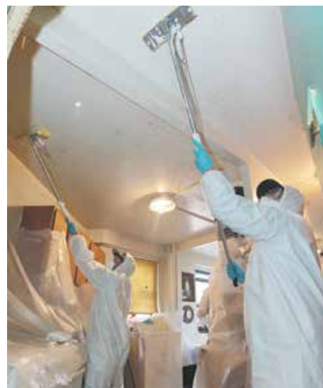
Internal repairs have been made at 24 developments in Coney Island, Red Hook, the Rockaways and Manhattan.
