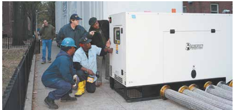
Fuel-efficient natural gas mobile boilers will save $22 million in energy costs over the next few years.
