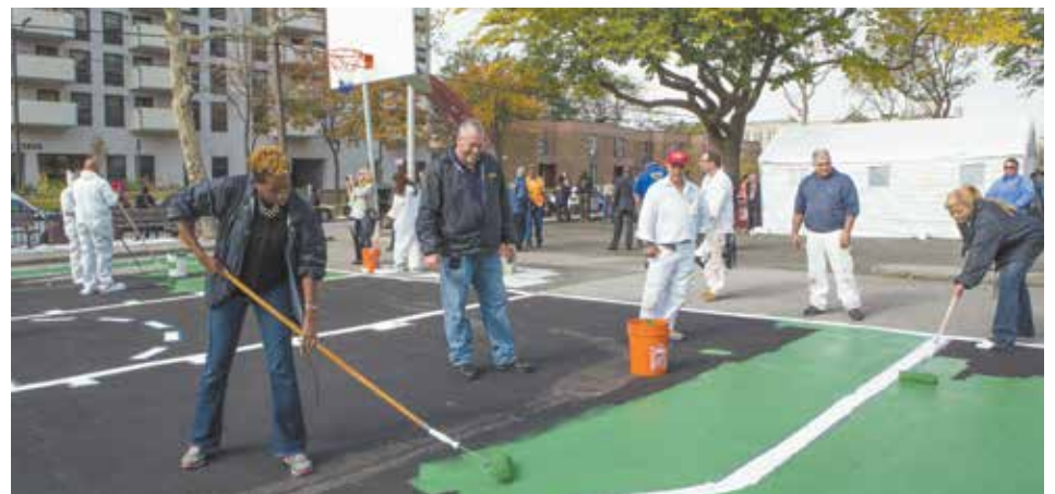
On October 29, 2014 NYCHA Chair Shola Olatoye, General Manager Cecil House, and NYCHA staff partnered with residents and community members at Carey Houses in Coney Island to repair and paint the basketball court and surrounding benches, install basketball nets, and plant more than 1,000 bulbs.
