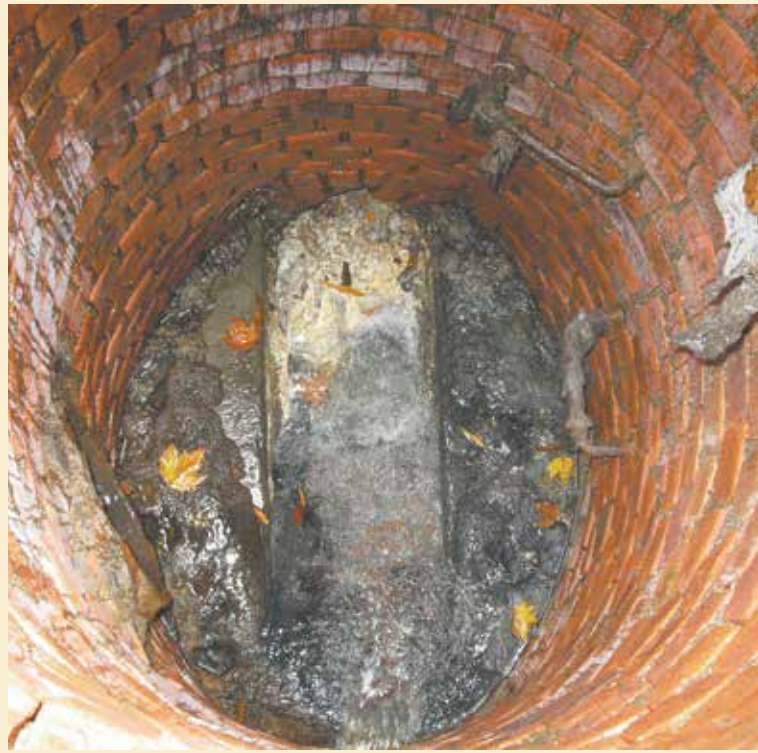
Grease build-up is shown in the sewer that services 70-72 Baruch Drive at Baruch Houses.
