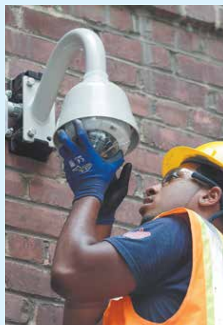
A NYCHA employee installs a CCTV security camera.
