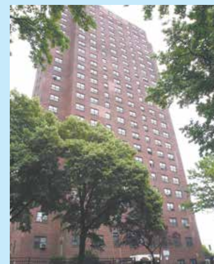
Kingsborough Extension is one of the first developments that will have repairs done with the $732 million in funding obtained by NYCHA through a new bond issuance.
