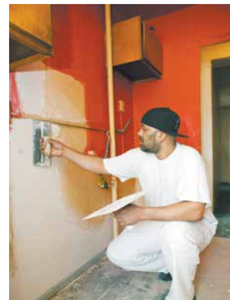
A NYCHA maintenance worker plasters a wall at Marble Hill Houses.
