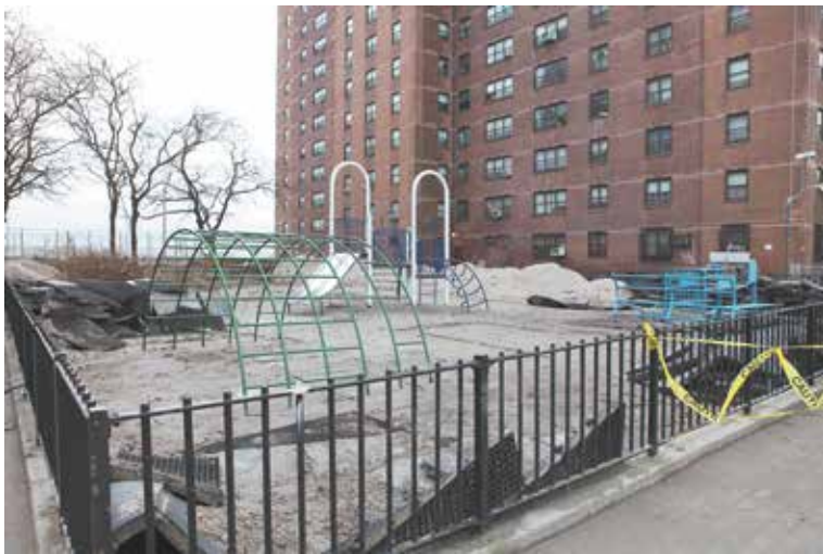
Hurricane Sandy damaged many playgrounds at NYCHA developments, including this one at Coney Island Houses.
