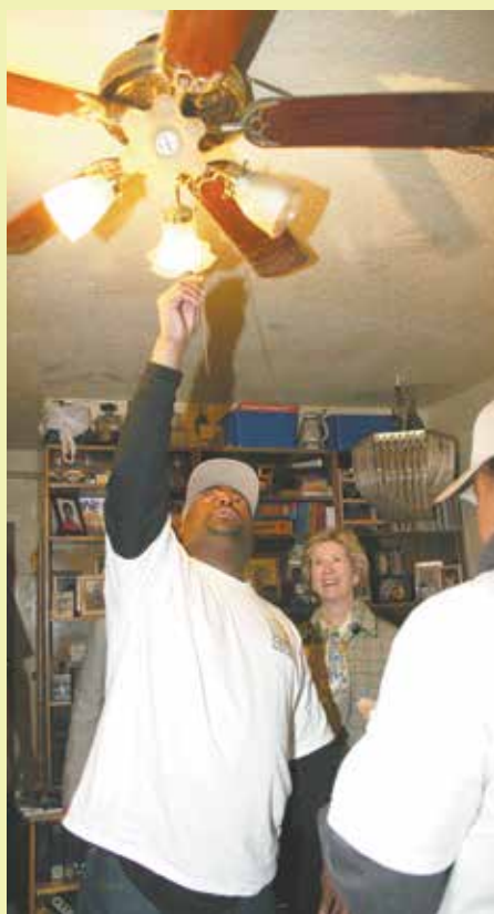
A NYCHA employee installs a free compact fluorescent lamp (CFL) at Queensbridge Houses.
