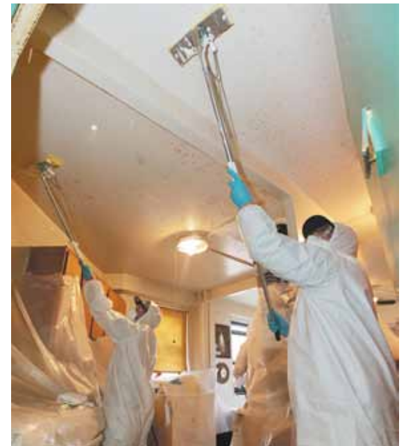
NYCHA contractors conduct mold remediation at LaGuardia Houses after Hurricane Sandy.
