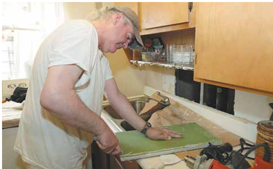
A NYCHA maintenance worker repairs a kitchen at Patterson Houses.
