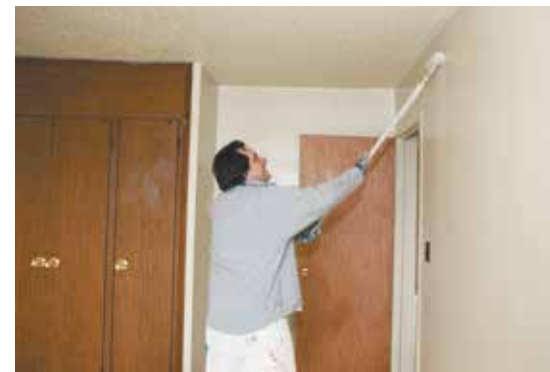
Despite $205 million dollars in cuts from the federal government as part of the sequester, NYCHA remains committed to eliminating its backlog of maintenance and repair work orders by the end of the year.
