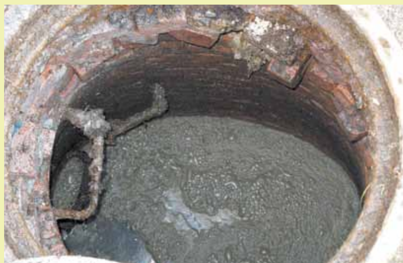
The grease that fills New York City's sewers can be seen rising up as NYCHA crews cleaned out the pipes near Baruch Houses on January 8, 2013. Photo by Daniel Osgood.
