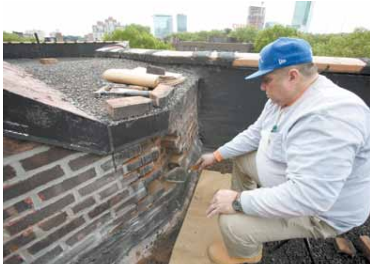
Part of NYCHA's capital repairs include fixing bricks and roofs.
