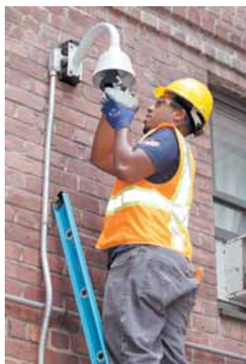
A new security camera being installed at Amsterdam Houses in Manhattan.
